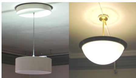
Lighting Upgrade: Before and After
