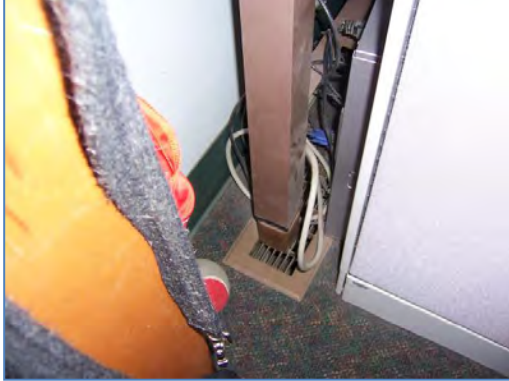
Partially blocked supply-air register in office area.
