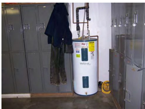
55g electric hot water tank in men's locker room
