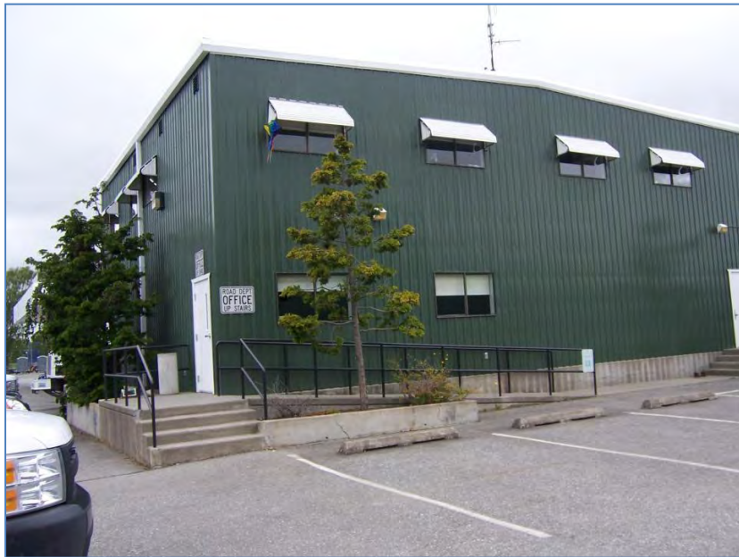
Skagit County Road Department Administration Building
