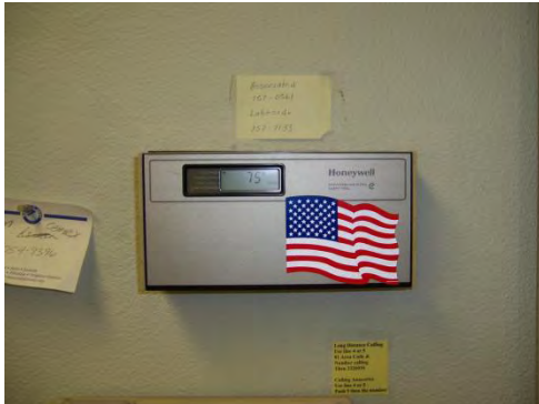
Thermostat in upstairs meeting room was set for cooling at 75 degrees. Temperature on the wall above thermostat and the walls surrounding the room was about 80! (Registers were delivering 75 degree air; outside air temperature was about 60 degrees!)
