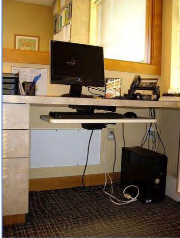
Photo shows 100W white infrared radiant heat panel that can be mounted under desk to help keep desk user comfortable.
