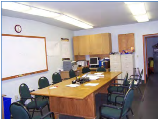
Significant heat gain is coming from ten 4-lamp overhead fluorescent fixtures – all on one switch. (When these lights are on, it's like having a 1500W personal space heater running in the room!)
