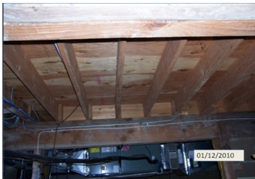
No insulation under ground floor of 2221 Riverside Dr.
