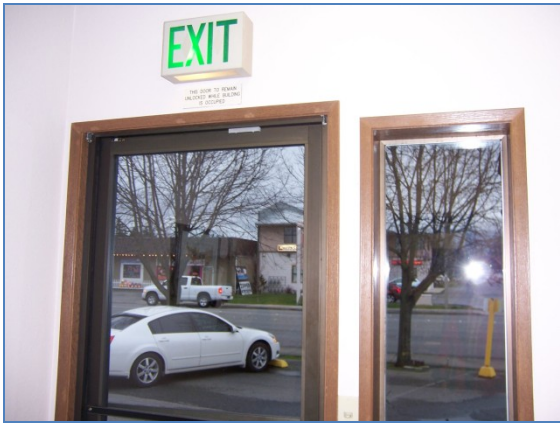
Apparent non-LED Exit Sign at 2221 Riverside Dr.
