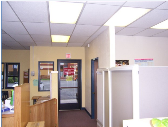
T-12 fluorescents in reception area at 330 Pacific Place
