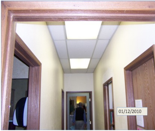
T-12 fluorescents in hallway at 2221 Riverside Dr.
