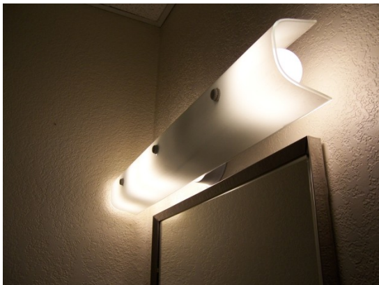
Incandescent bulbs above vanity in Men's restroom at 330 Pacific Place.
