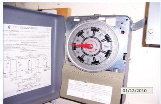
There is a night setback timer for HVACs at 330 Pacific Place, however Facility Maintenance staff were unsure how to use it and all pins controlling the timers were removed.
