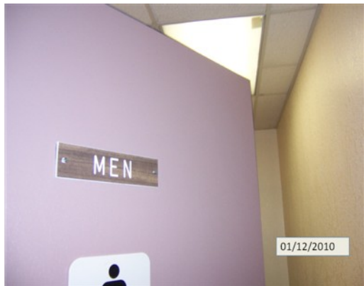
Unoccupied Men's restroom with overhead and vanity lighting turned on at 330 Pacific Place.
