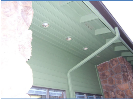
Incandescent outside lighting at 2221 Riverside Dr.
