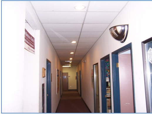
Incandescent lighting in hallway at 330 Pacific Place.
