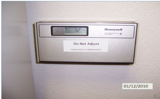
72 degrees in occupied offices at 330 Pacific Place.
