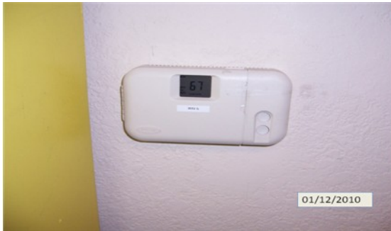
Some thermostats control registers in diverse spaces with different heating/cooling needs, such as this one at 320 Pacific Pl. for an office area, conference room & bathroom.
