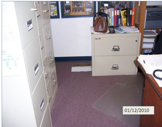
Occupants sometimes cover registers to keep rooms from getting too warm/cold, such as this one at 330 Pacific Place.
