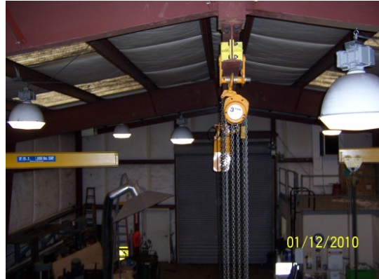
This is especially important where there are several 400W overhead lights turned on, such as the Maintenance Shop.
