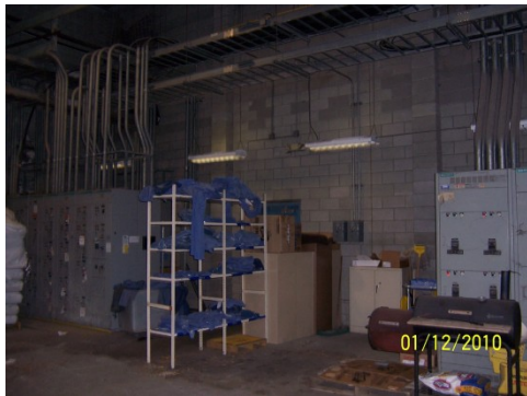
Linear fluorescent overhead lighting left on in unoccupied Sweeper storage room.
