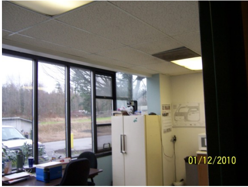
Lighting left on in unoccupied break-room. (natural lighting may be fully sufficient at times)
