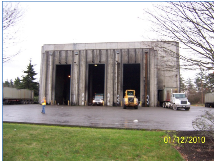
Ovenell Transfer Station - Commercial Waste Receiving Area
