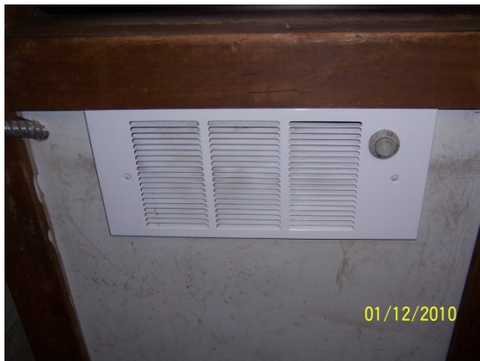
Electric wall heater in Scale House
