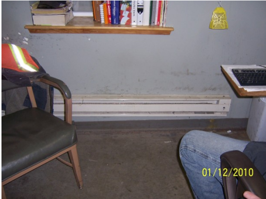
Baseboard heaters in Haz. Waste Bldg Office.
