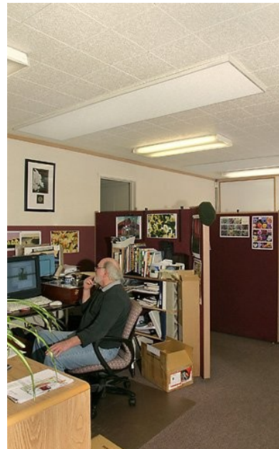
Example of infrared radiant heat panels on ceiling in office area.
