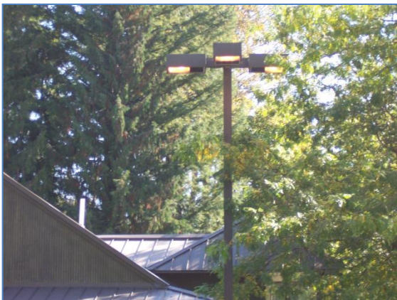
Several parking lot lights were observed on at 10 am on a bright sunny day.
