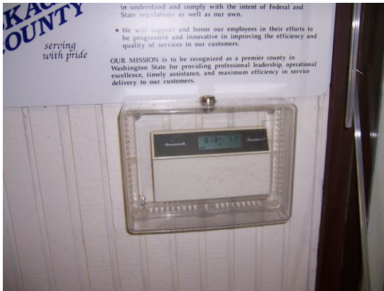
Locked cover on main thermostat
