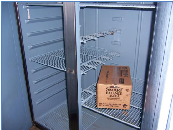
Delfield 2-door reach-in commercial refrigerator was nearly empty
