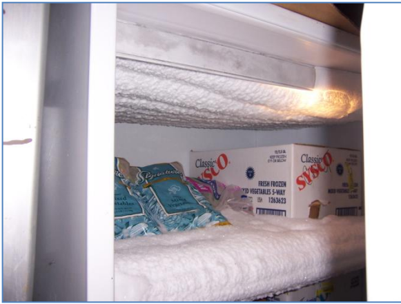
Large buildup of ice in this upright freezer
