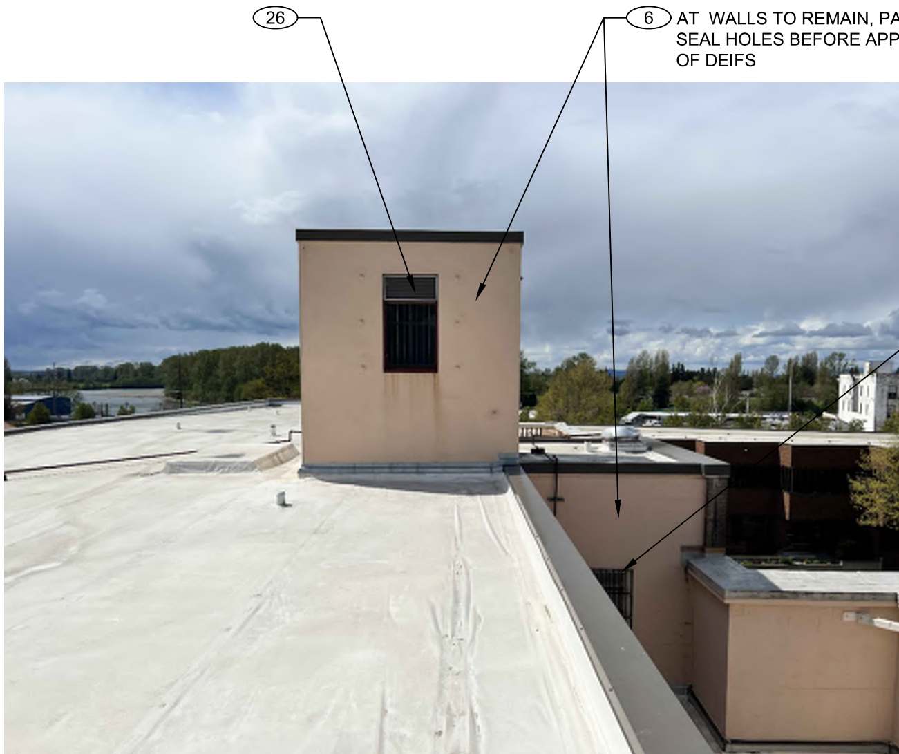
26 BASE OF ELEVATOR TOWER AND JAIL ROOF A0.5 NOT TO SCALE
