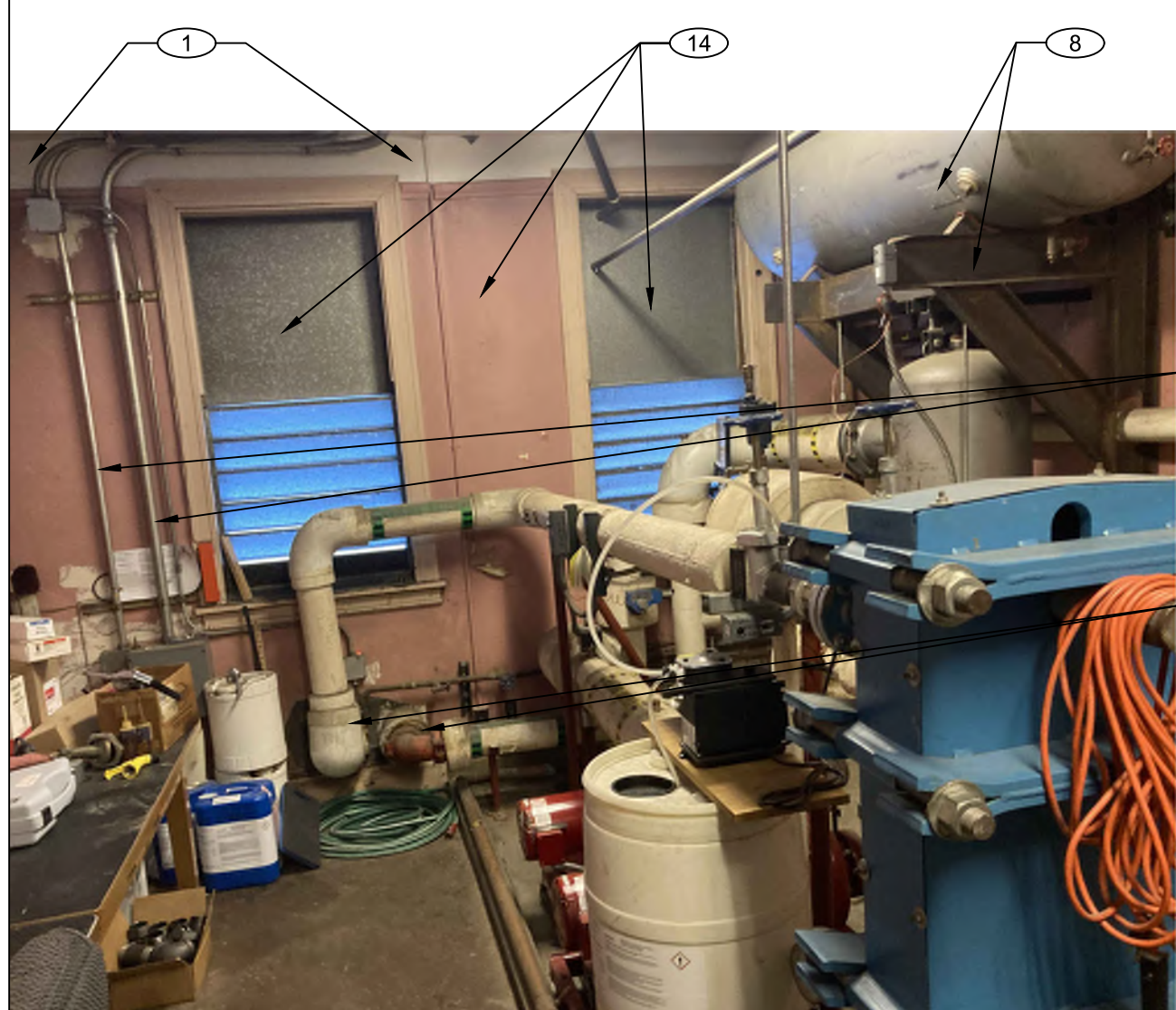
10 MECHANICAL ROOM FACING NORTH A0.4 NOT TO SCALE
