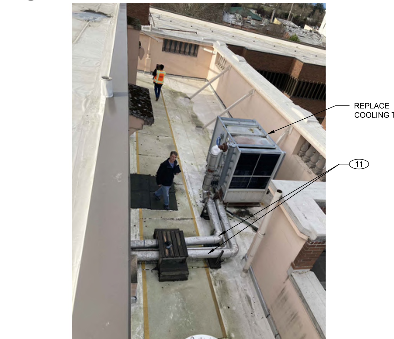
17 COOLING TOWER NORTH A0.4 NOT TO SCALE
