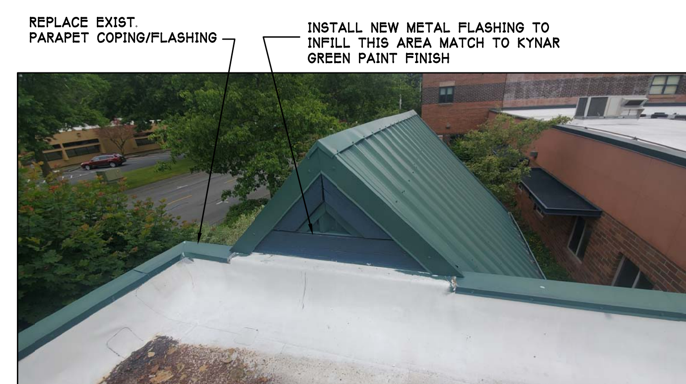
7 EXISTING ROOF TO WALL FLASH COUNTER FLASHING N.T.S.
