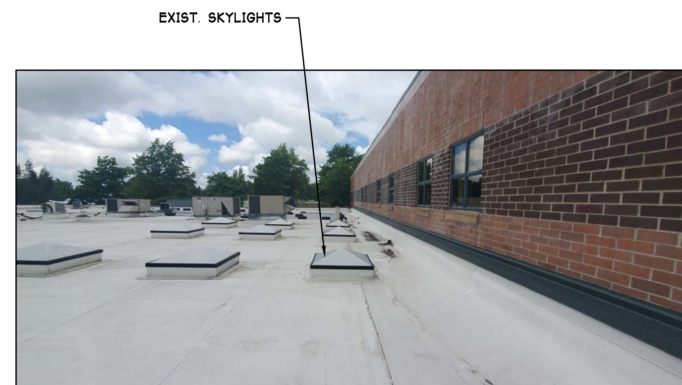
5 SKYLIGHT LOOKING WEST
