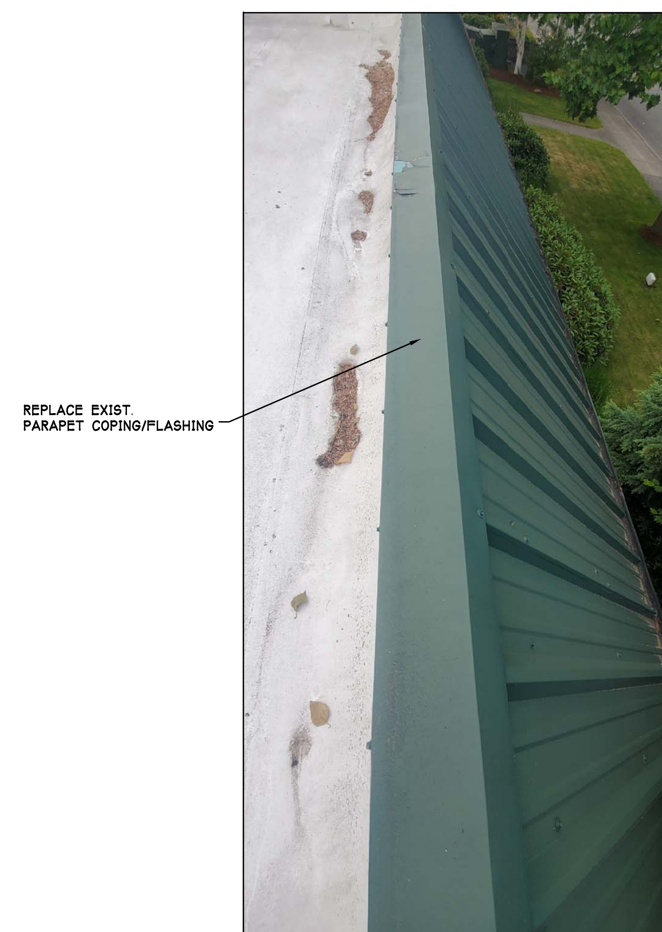
7 EXISTING ROOF TO WALL FLASH COUNTER FLASHING N.T.S.
