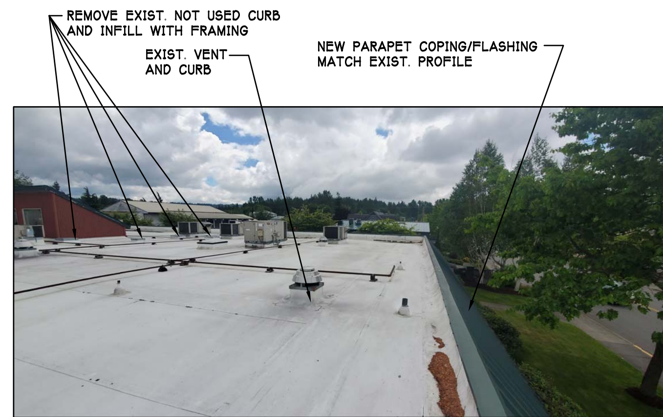
14 MANSARD PARAPET FLASHING
