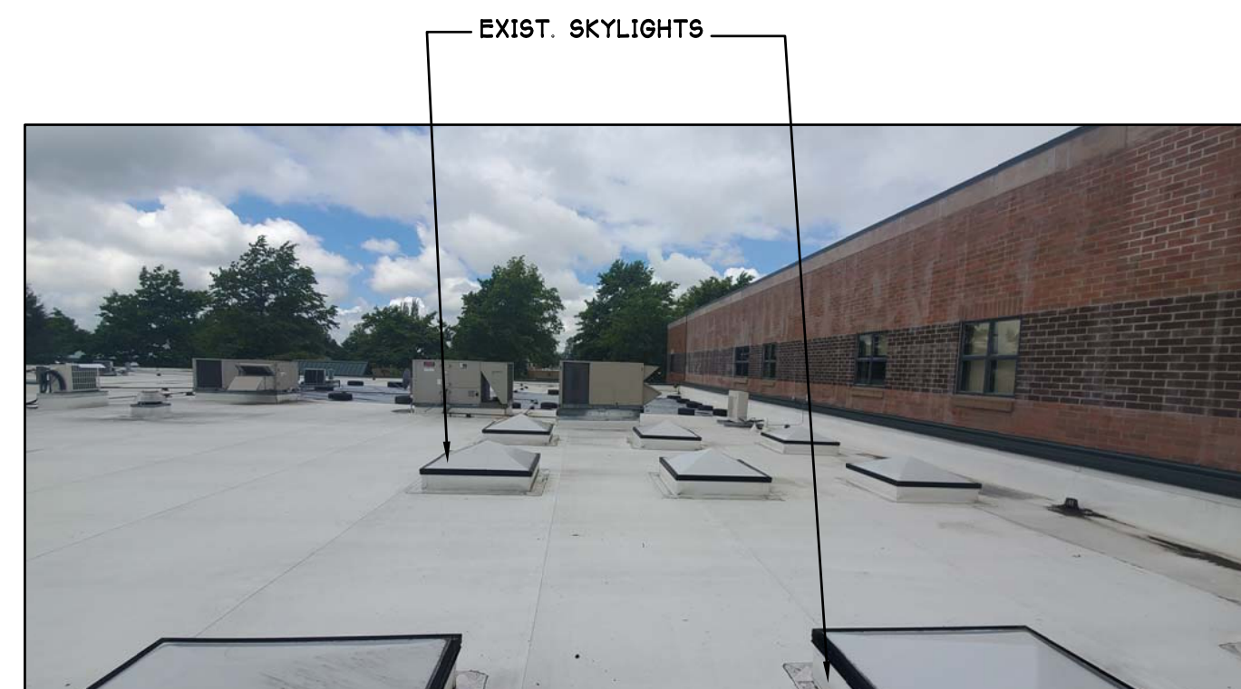
8 VIEW LOOKING WEST SKYLIGHTS
