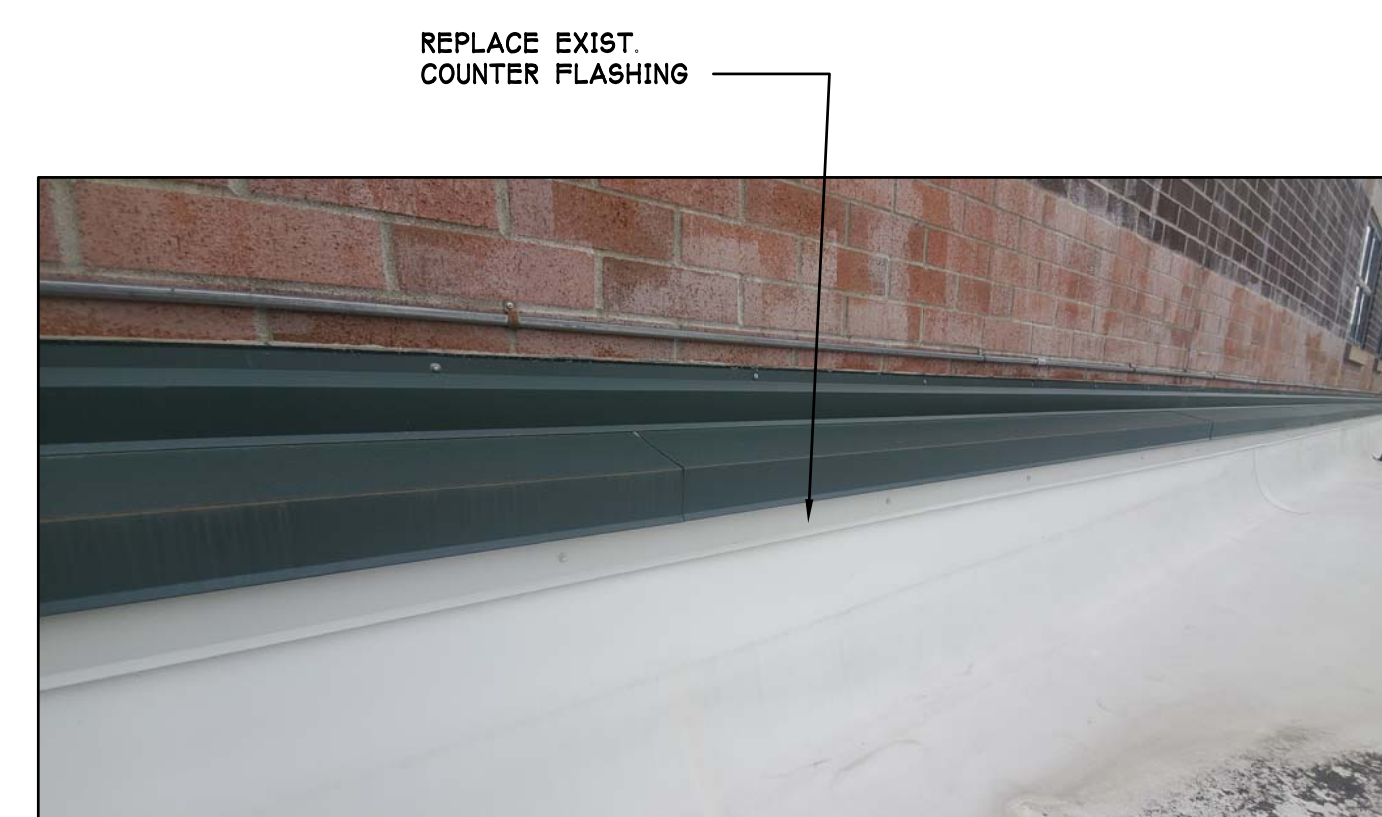
7 EXISTING ROOF TO WALL FLASH COUNTER FLASHING N.T.S.
