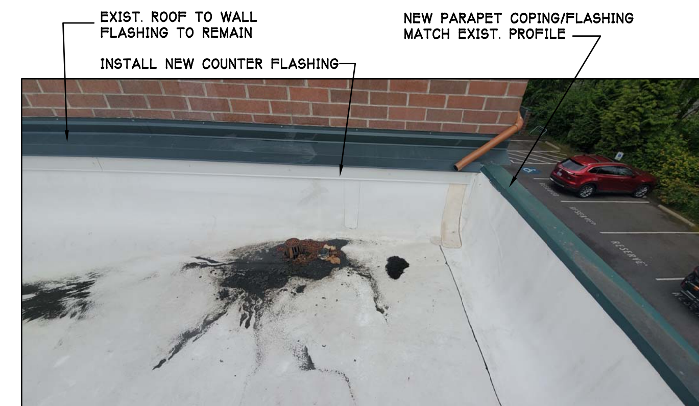
4 ROOF DRAIN/OVERFLOW NE CORNER ROOF TO WALL FLASHING
