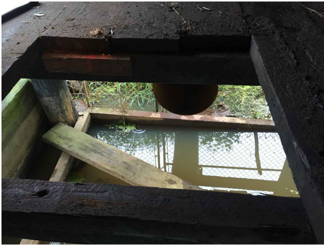
FLOOR OPENING AND EXISTING 18-IN DISCHARGE PIPE
