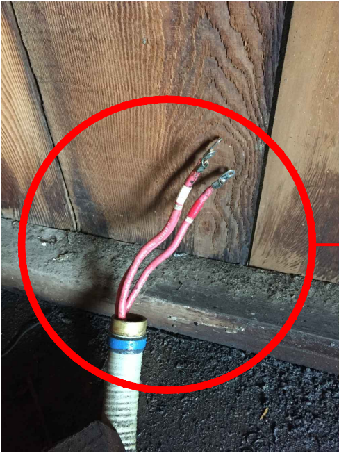
EXISTING ELECTRICAL CONNECTION FOR PUMP MOTOR
