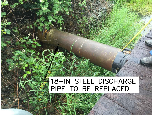
18-IN STEEL DISCHARGE PIPE
