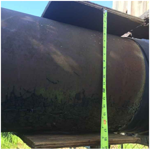
EXISTING DISCHARGE PIPE SIZE
