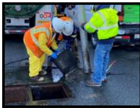
Figure 10-1. A crew replaces a stormwater filter in a catch basin at near Guemes Island Ferry Terminal
