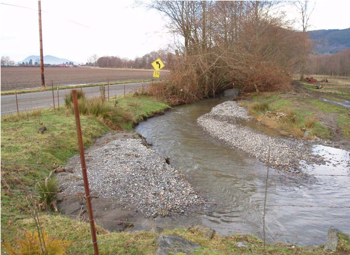
Photo 3. Viewing downstream from the crossing at Colony Mountain Road.
