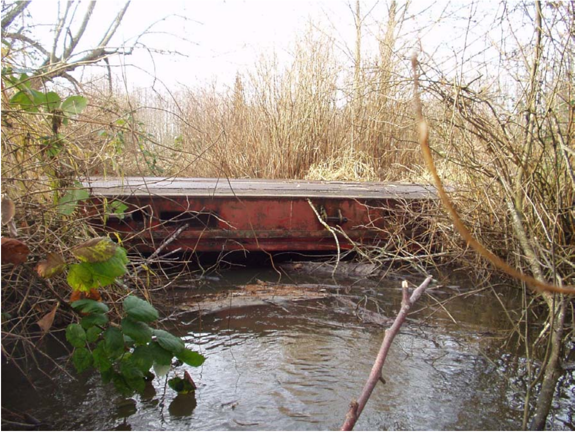
Photo 5. Viewing west to the downstream driveway bridge near the downstream end of the project reach. Water is nearly stagnant and bed material here is mucky silt.
