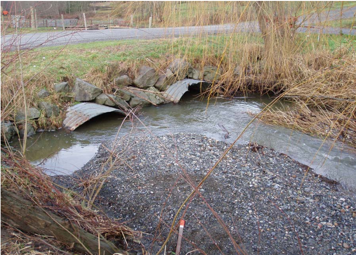
Photo 2. Viewing downstream to the entrance to the culverts under Colony Mountain Road.
