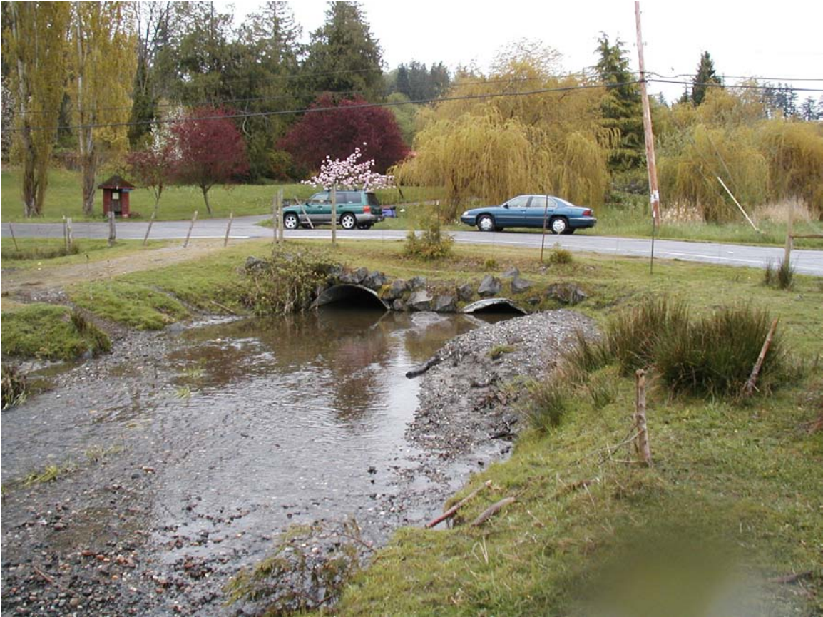
Photo 1. Viewing upstream (east) to the twin 7-ft diameter CMP culverts under Colony Mountain Road.
