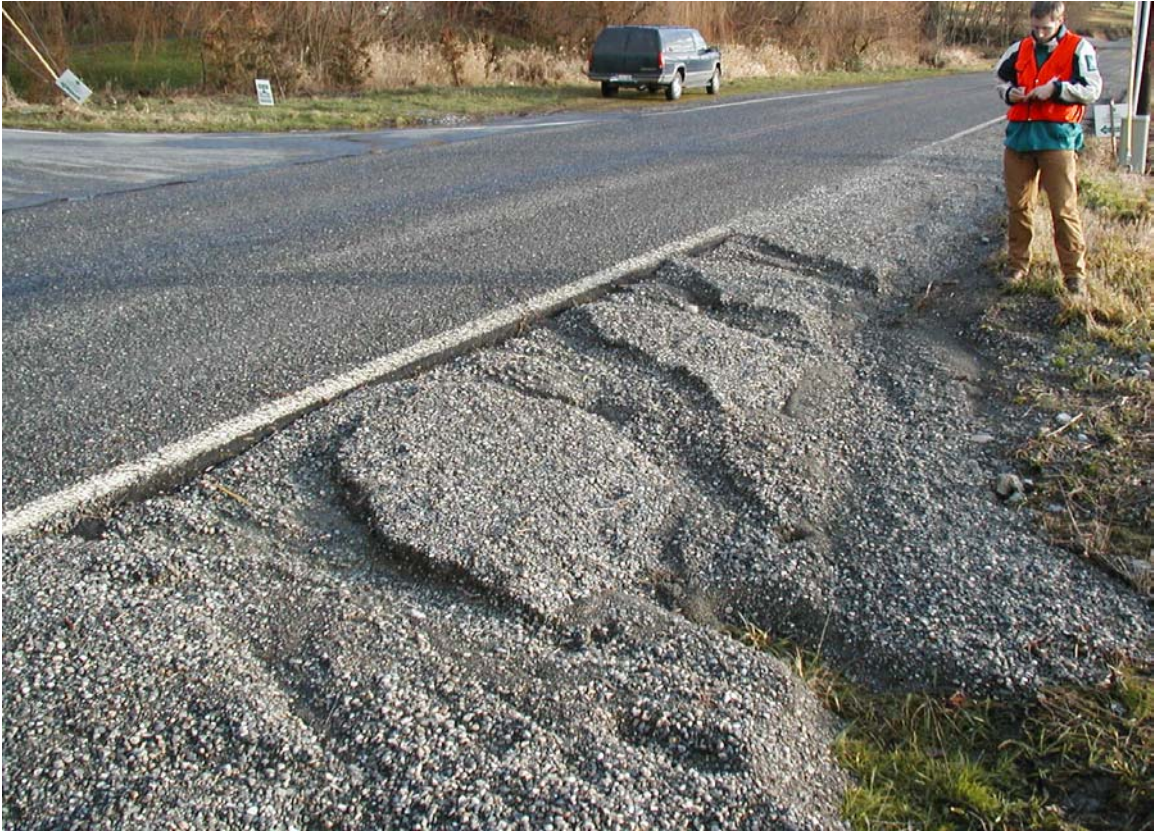
Photo 7. Erosion scars along the south edge of Colony Road at Colony Mountain Road. Scars were caused by water ponding upstream of the culverts and overtopping the road during the January 3, 2007 flood.
