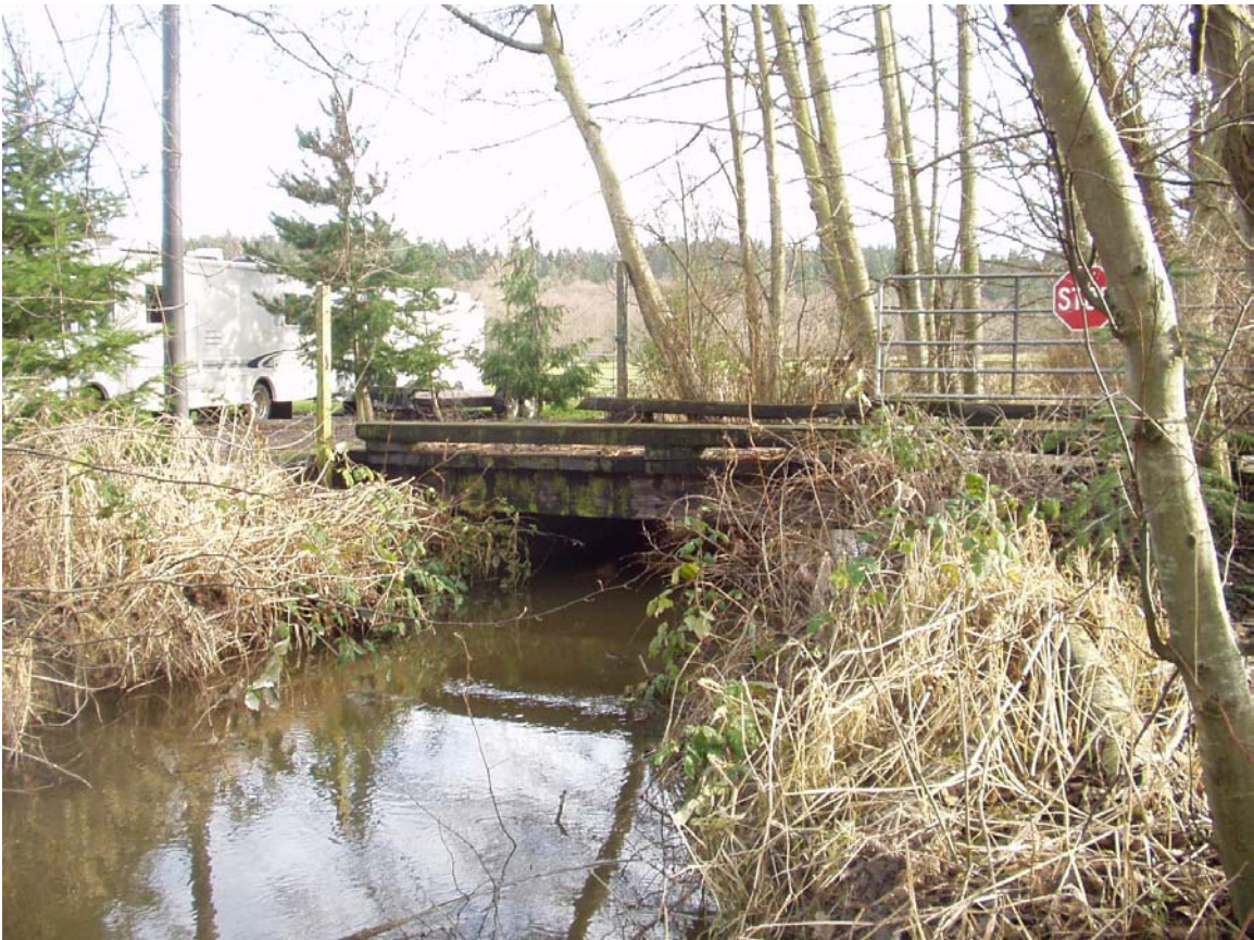
Photo 4. Viewing east to the upstream driveway bridge near the downstream end of the project reach. Water is nearly stagnant and bed material here is mucky silt.
