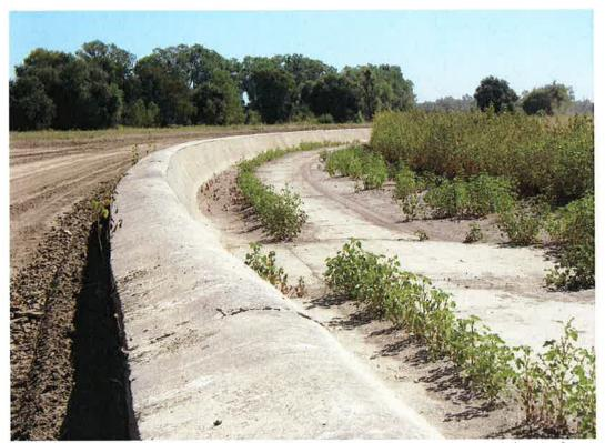
Two styles of passive overtopping weirs which have been used in California for years. Top: Fremont weir is 1.9 miles long and functions in a 340,000 cfs river system. Bottom: Tisdale weir capacity is 38,000 cfs. Flow is limited by length/elevation and could be designed to provide 2 to 10 year flood protection for Nookachamps basin.
