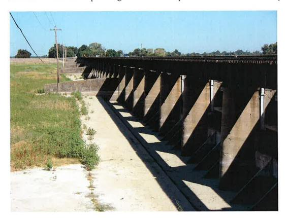
2,500' Corps designed gated outlet structure, capacity 110,000 cfs, on Sacramento River. 25 individual gates can be operated independently for flow control. Could control filling/evacuating of Nookachamps storage when located directly upstream of BNSF Bridge. Existing levee would be removed and basin flood water evacuation improved.
