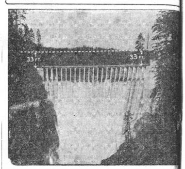
With 33 feet added to the height of the Baker River Dam at Co for the Puget Sound Power & Light Company the great structure be 293 feet high, practically doubling the water storage capacity.
