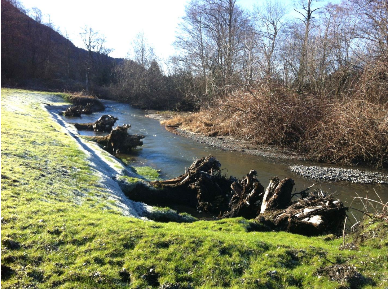
NRSP has installed 100 pieces of large woody debris through landowner projects since 2009; plantings later installed on the bank help prevent erosion
