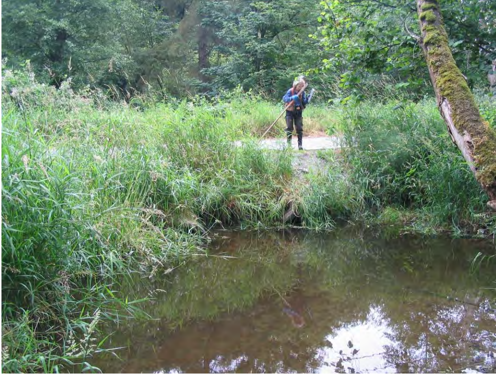
Figure 42. Bulson Road Culvert Crossing
