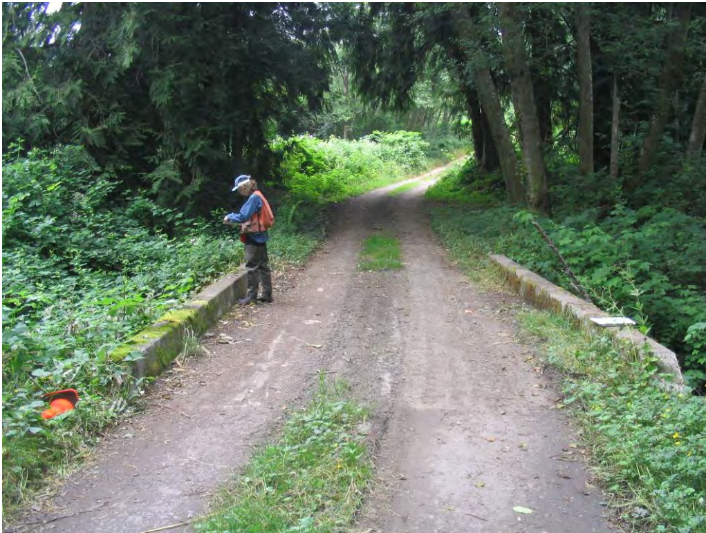
Figure 40. Bridge crossing N. Fork Bulson Creek on Sixteen Lake Camp Road
