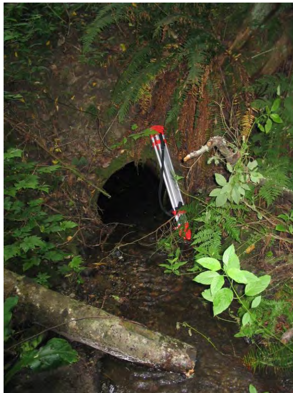
Figure 35. Bulson Creek, Upstream side of West English Road Culvert
