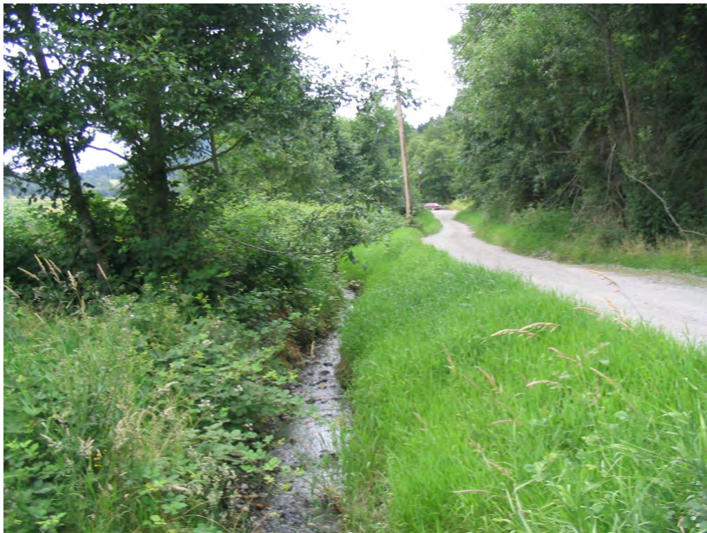
Figure 17. Looking at Sandy Creek/Hill Ditch confluence at Kanako Road Bridge
