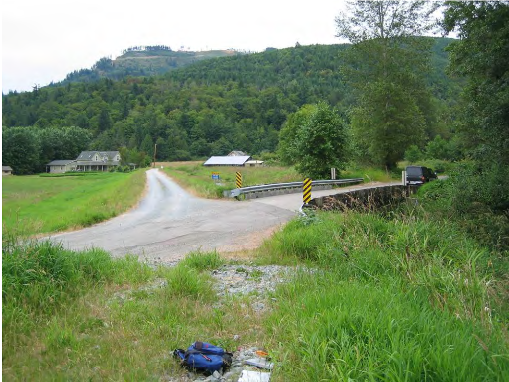
Figure 28. Looking north along levee towards Johnson Road bridge
