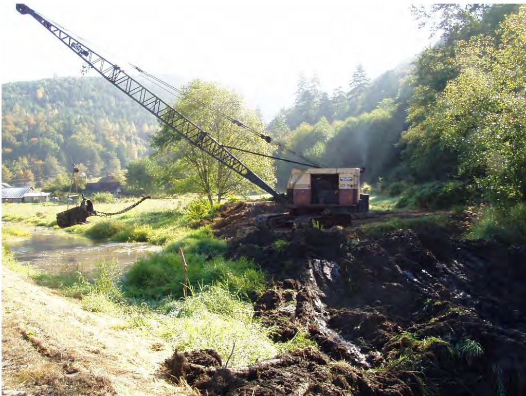
Figure 29. September 2006 dredge operations at mouth of Johnson Creek
