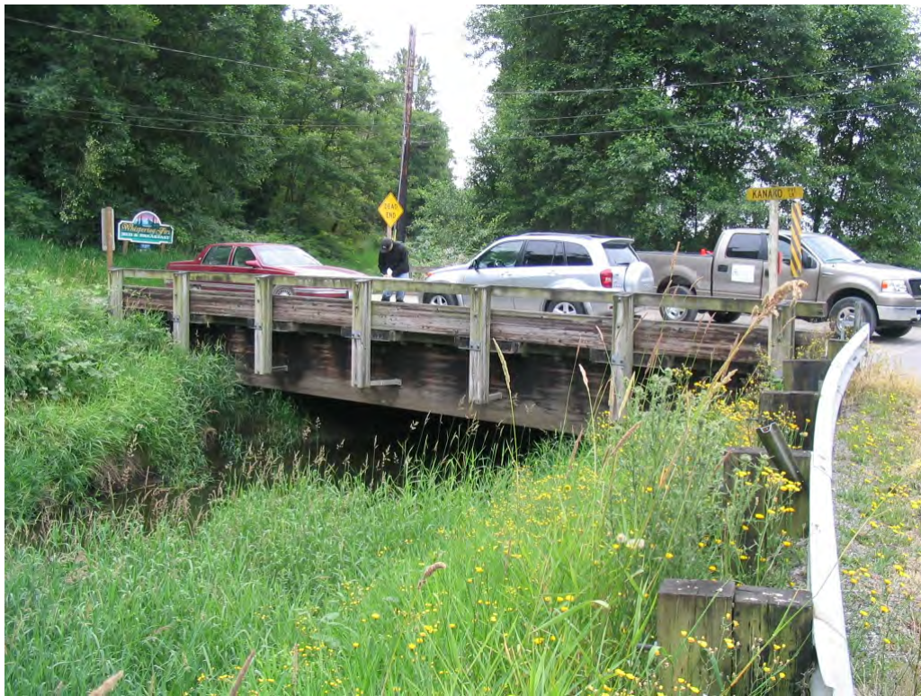
Figure 18. Looking at Sandy Creek/Hill Ditch confluence at Kanako Road Bridge
