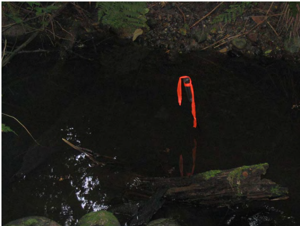
Figure 36. Bulson Creek, Downstream side of West English Road Culvert, fully submerged and partially blocked with debris
