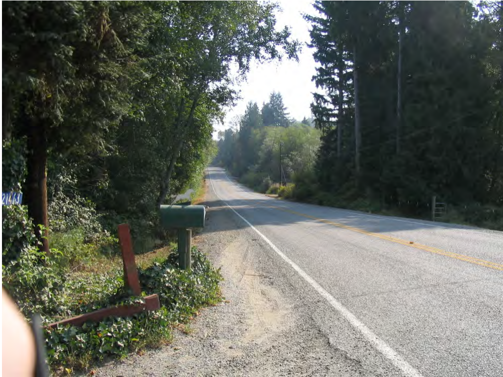
Figure 7. Little Mountain Road looking towards problem culvert area near Lang Pony Farm driveway
