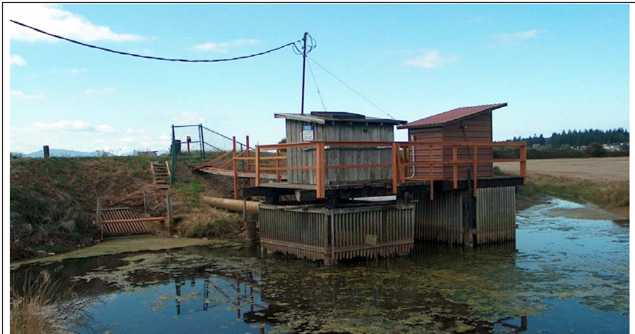
No Name Slough Outfall and Pump Stations
