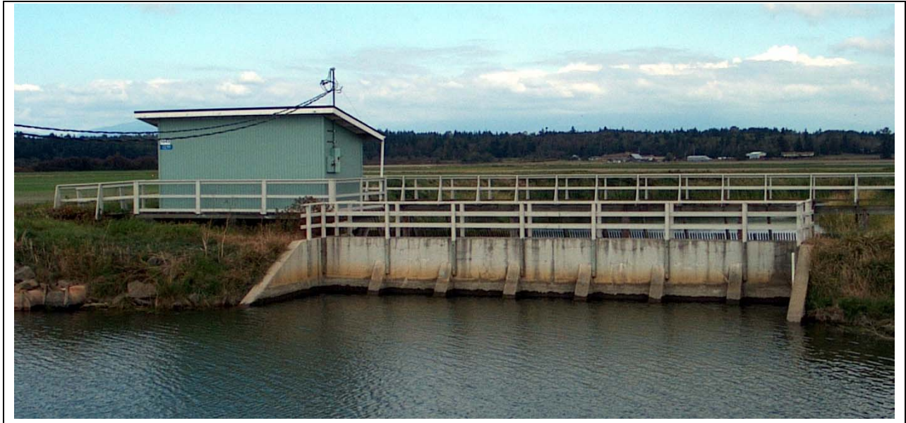
Big Indian Slough Outfall and Pump Station
