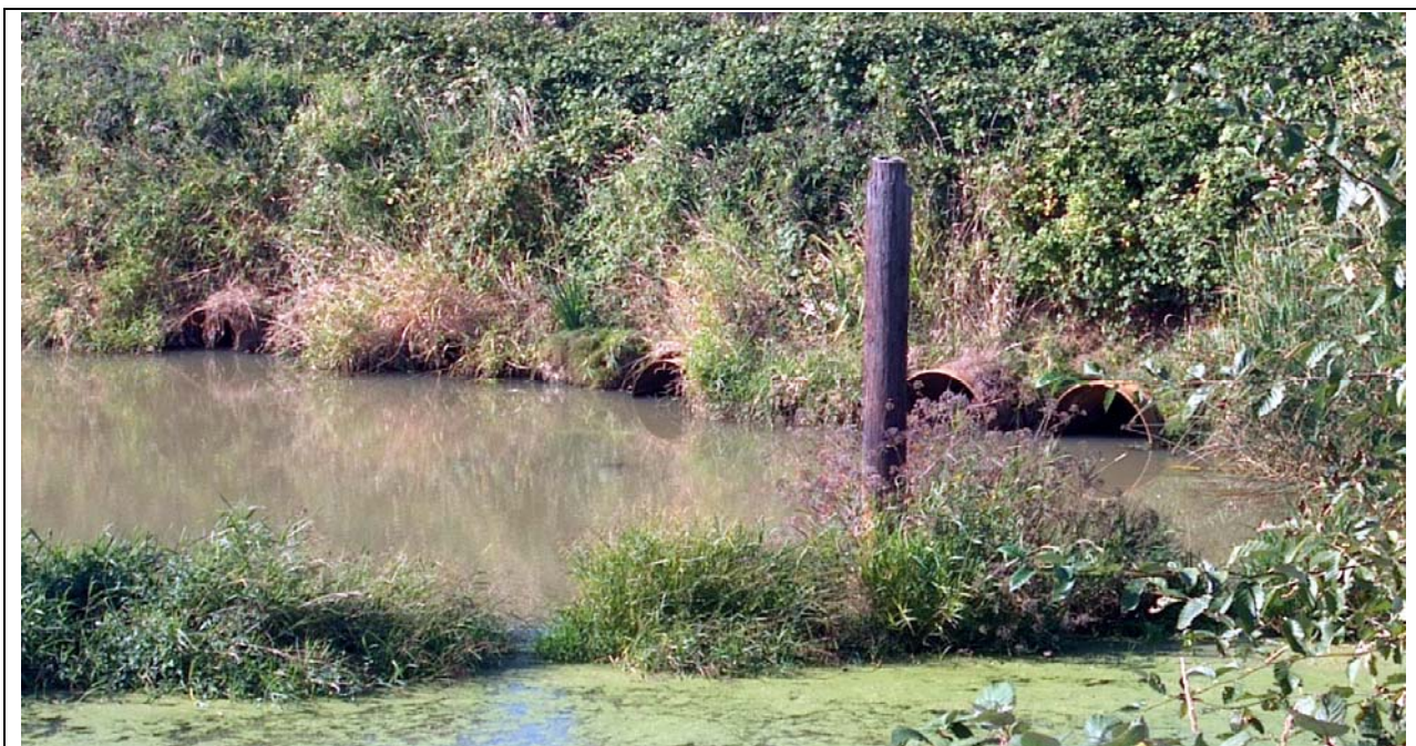
Joe Leary Slough Outfall
