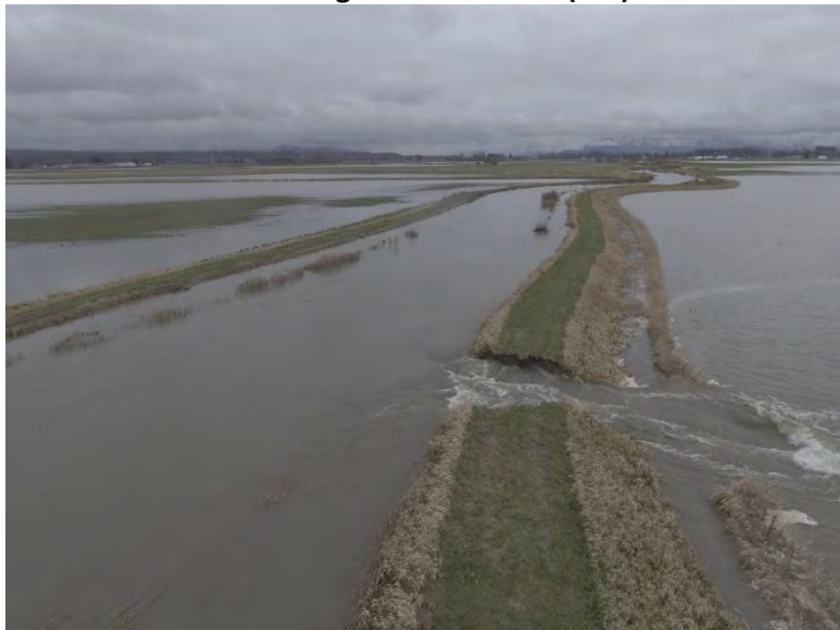
Photo A2.5 Photo from UAV looking at Samish River dike breach, taken February 6, 2018 – courtesy of Austin Breckenridge. (left)
