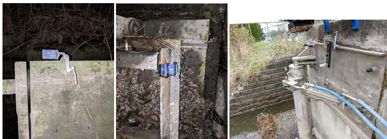
Figure 2.2 Gate Position Sensors and downward looking trail camera (top hinged gates left and center; SRT control arm at right)
