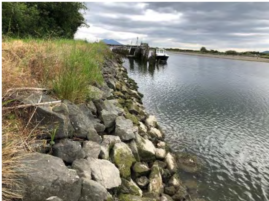
Photograph 2. The Bayview Edison North levee is armored with rip rap and supports a timber pile pier structure.
