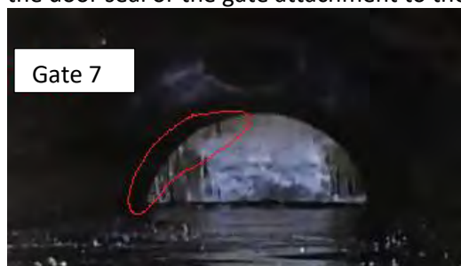
Figure 2.10 Leakage through top of Gate 7 (from video DSCI16004.MOV)
