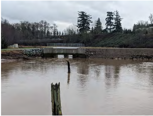
Photo I12.1 Joe Leary Slough Side Hinge Tide Gates, Installed in Summer 2019
