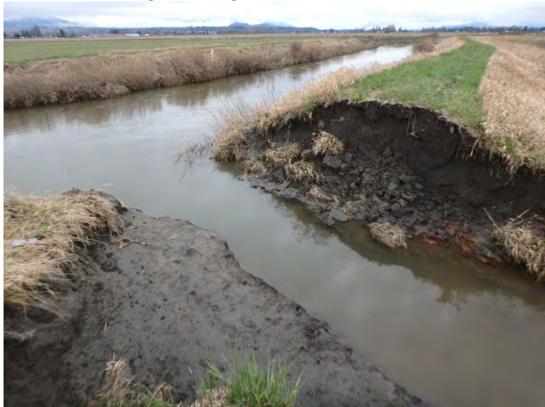
Photo A2.3 Post flood photo of Samish River dike breach, looking toward river, taken February 15, 2018 following flood recession (left)
