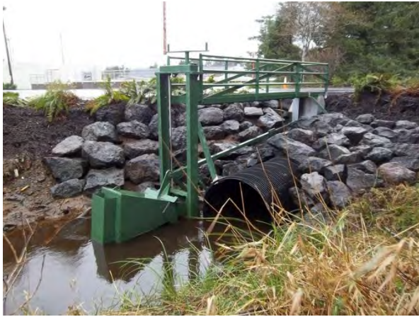
Photo I12.6 Examples of MTR tide gates. Left: unknown location; Right: Fisher Slough (Pictures from http://www.nehalemmarine.com )
