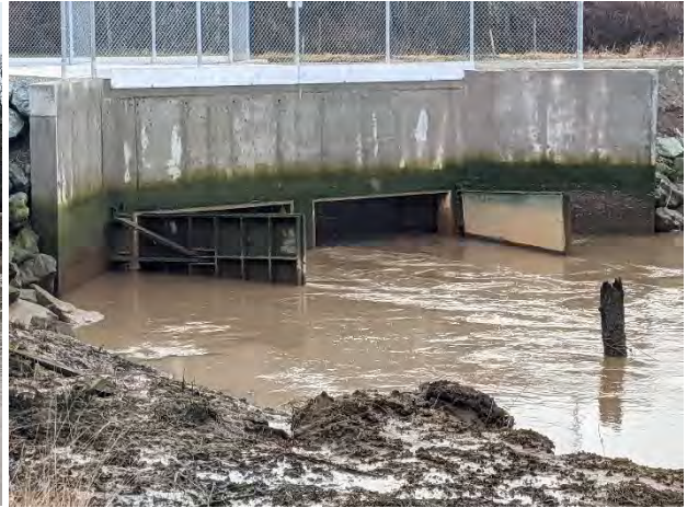
Photo I12.1 Joe Leary Slough Side Hinge Tide Gates, Installed in Summer 2019
