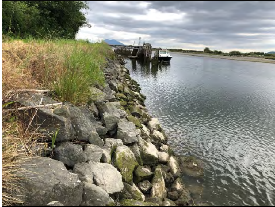
Photograph 5. The Bayview Edison North levee is armored with rip rap and supports a timber pile pier structure.
