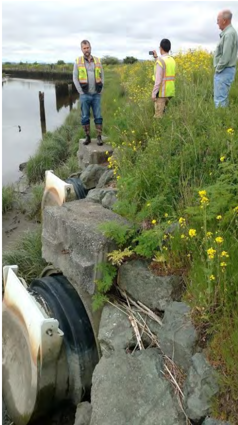
Photo A.6 Existing Bayview Edison South Flood Relief Structure Outlets
