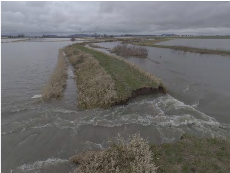
Photo A2.5 Photo from UAV looking at Samish River dike breach, taken February 6, 2018 – courtesy of Austin Breckenridge. (left)
