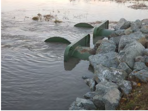
Photo I12.4 Farm to Market Replacement with Side Hinged Tide Gates (left)
