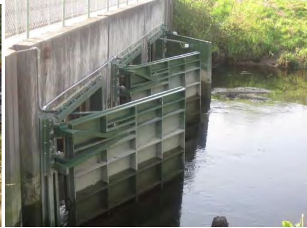
Photo I12.6 Examples of MTR tide gates. Left: unknown location; Right: Fisher Slough (Pictures from http://www.nehalemmarine.com )
