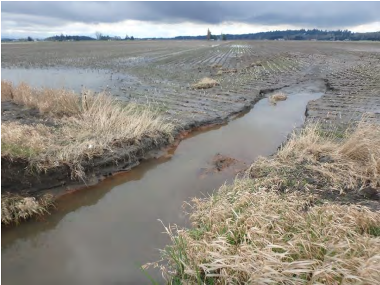
Photo A2.3 Post flood photo of Samish River dike breach, looking toward river, taken February 15, 2018 following flood recession (left)
