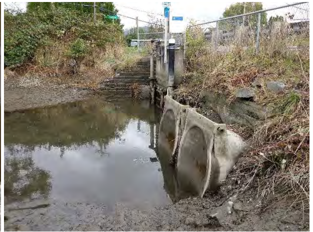
Photo I12.5 Left: Top view of Edison Slough SRT gate. Right: Side view of traditional top-hinged gates (near) and SRT gate (far) at Edison Slough
