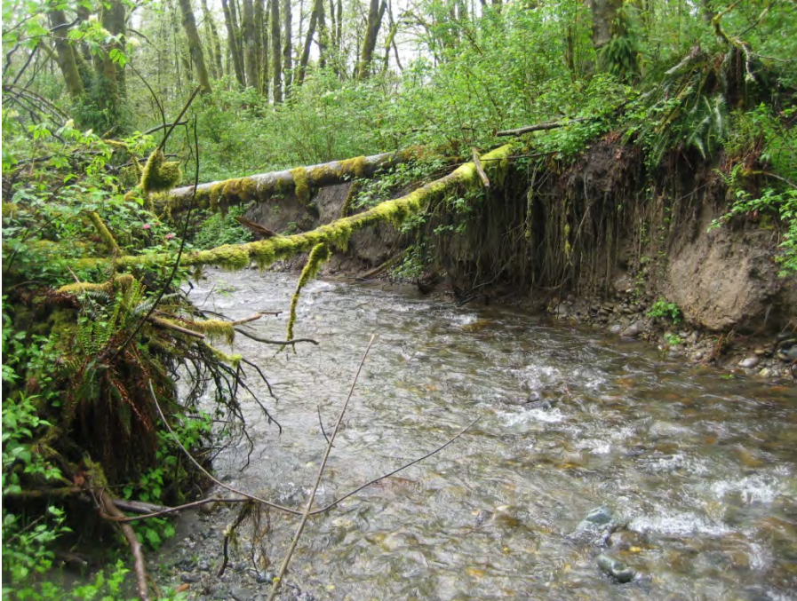
Picture 5. Large eroded bank on right-bank near end of intensive habitat survey (Reach K). Active erosion and sediment recruitment including several recently fallen trees with green leaves. Bank is approximately 30 feet high and 100 feet long, with undercutting of alder trees at the top of the bank.
