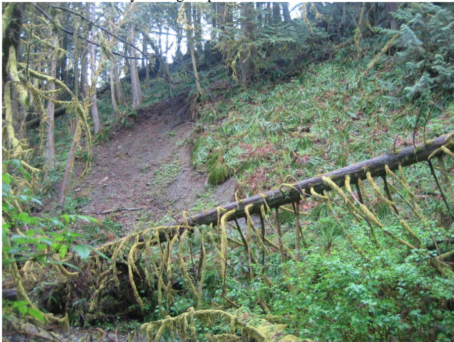
Picture 13. Currently failing slope with indication of historic failure.
