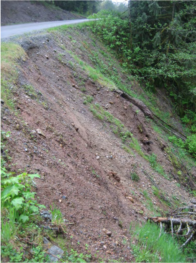
Picture 14. Active erosion that is possibly human caused, near horse camp bridge.
