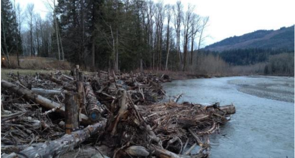
Figure 9. An engineered, complex wood revetment built by the Lummi Nation along the South Fork Nooksack River. The structure is stabilized with timber piles and rock collars creating a rough streambank very different than traditional rock revetments such as riprap.
