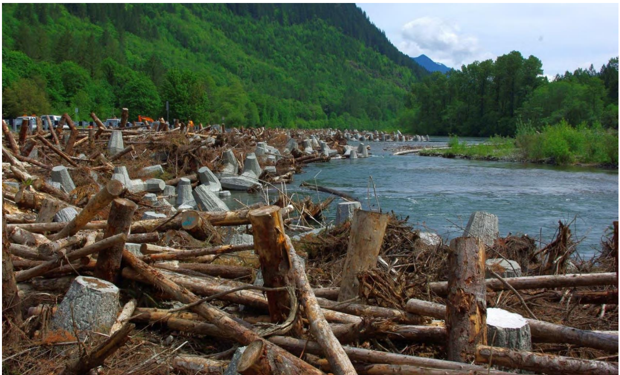
Figure 10. An engineered, complex wood revetment constructed by WSDOT on the Skagit River to protect SR 20 at milepost 100.7. This structure is stabilized with concrete dolo anchors and ballast due to site constraints. Photo from WSDOT (2014).
