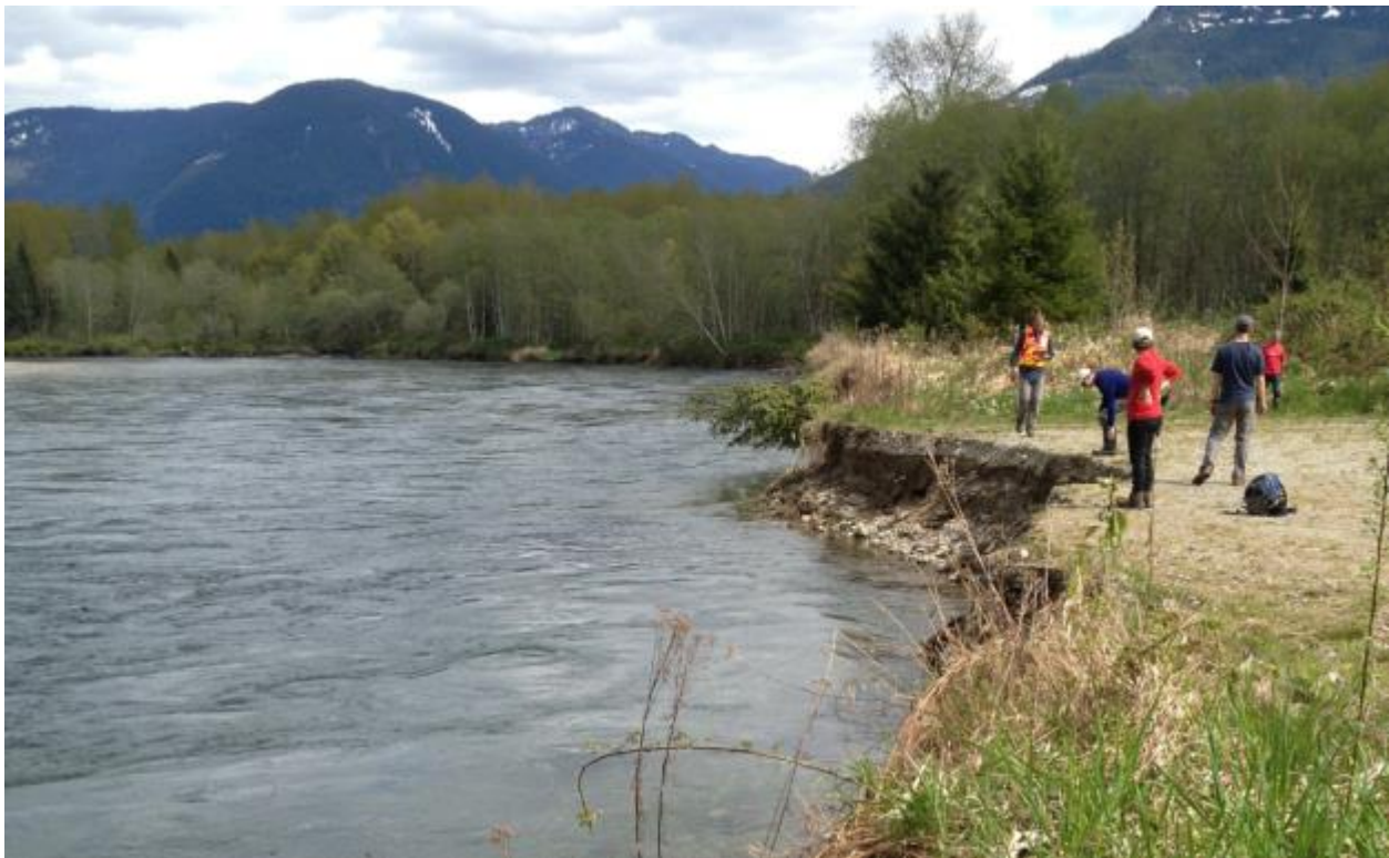
Figure 4. Photo looking upstream along eroding (left) bank at the WDFW access site near the 90 degree bend in Martin Road.
