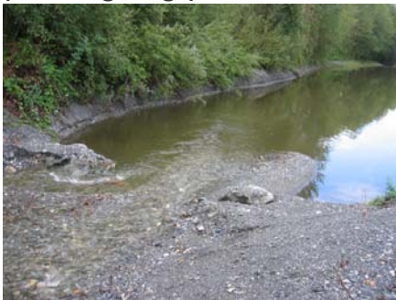
Photo D4: Minkler Road sediment trap (looking upstream) with the recent installation of LWD designed to maintain sediment transport through this reach and into the depositional area (following image)
