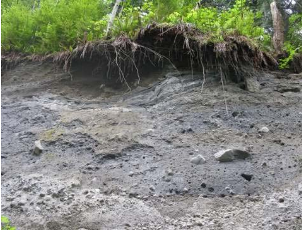
Picture 9. Eroded bank – looking up the hill-slope showing severe erosion and undercutting of mature vegetation.
