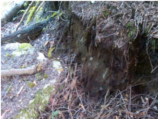
Photo D11: Evidence of recent slope instability
