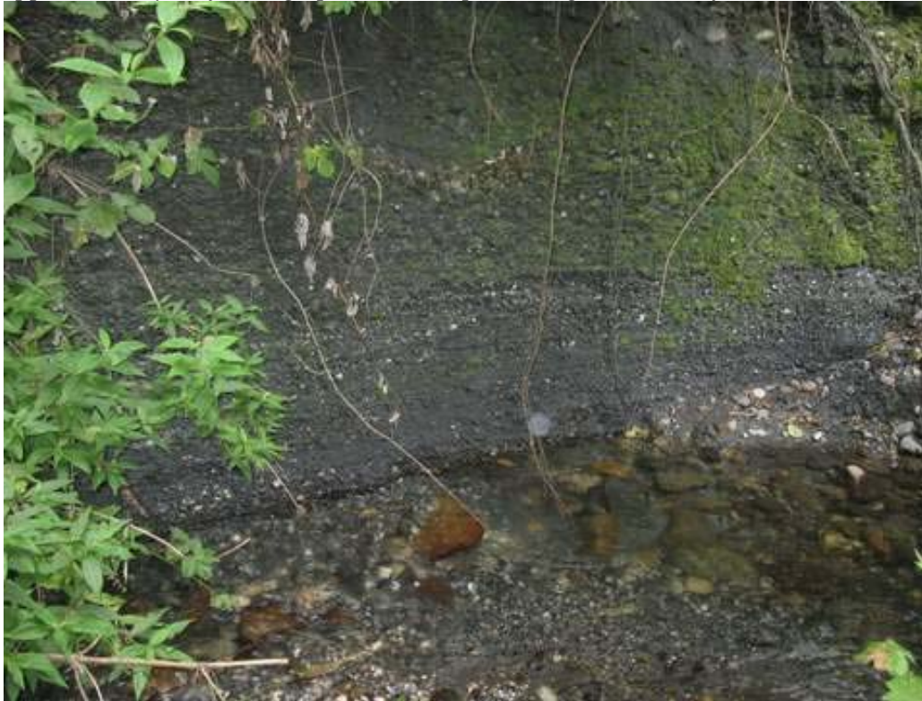
Picture 12. Left-bank erosion and sediment source exists as a tall, flat “wall” of sediment approximately 10 feet high packed with pebbles, gravels, and fines. Active sediment recruitment.
