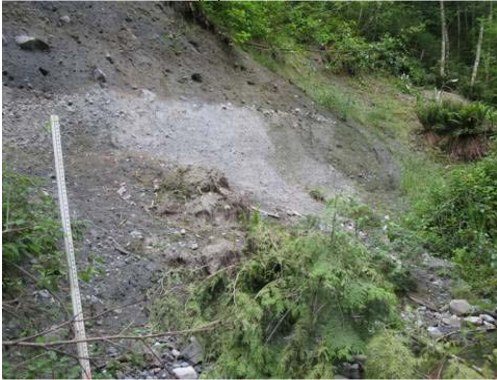
Picture 6. Eroded bank looking upstream.
