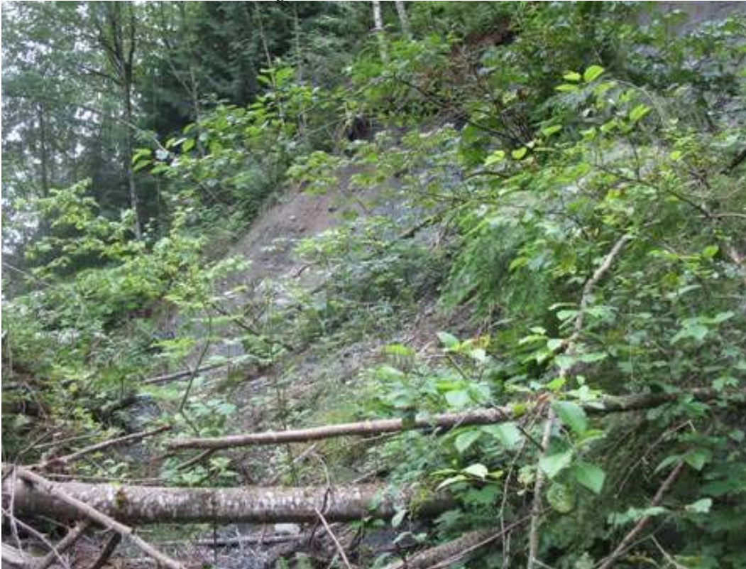
Picture 7. Eroded bank looking downstream.
