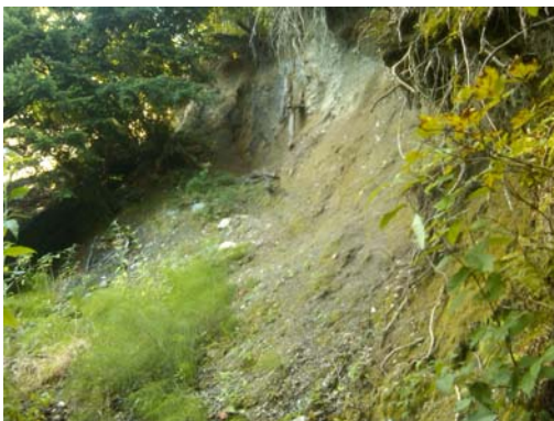
Photo D12: Evidence of recent slope instability
