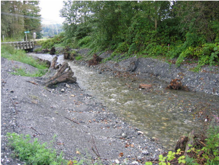
Photo D4: Minkler Road sediment trap (looking upstream) with the recent installation of LWD designed to maintain sediment transport through this reach and into the depositional area (following image)
