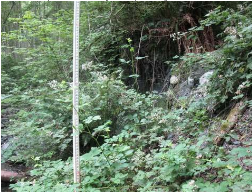
Picture 10. Left-bank erosion upstream from large eroded bank.
