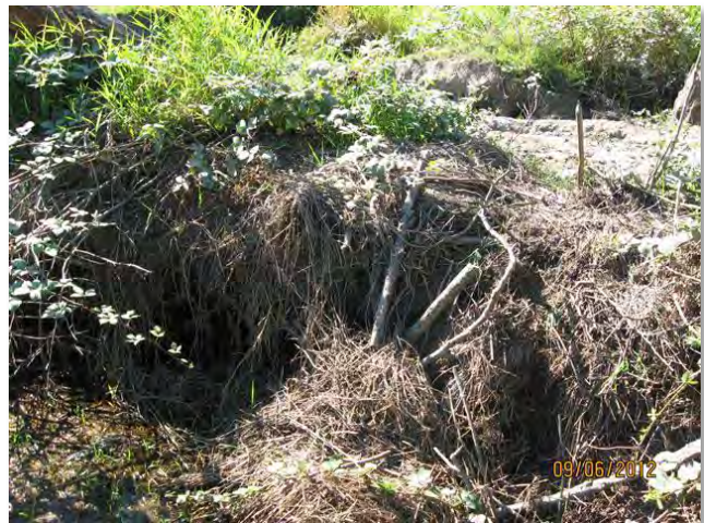
Figure 10. Partially plugged culvert (RM 0.04)
