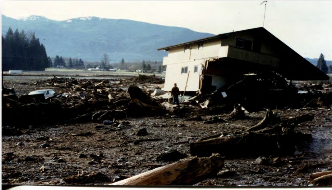
Photo 2: Hamerski residence, 1983. The house was unoccupied at the time it was impacted by debris and transported 100 feet downstream of its foundation. In the same storm event, a debris flow fatality occurred in Skagit County near SR 9.
