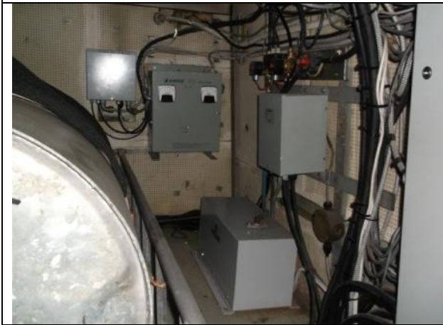
15 Potable Water Tank & Battery Charger
