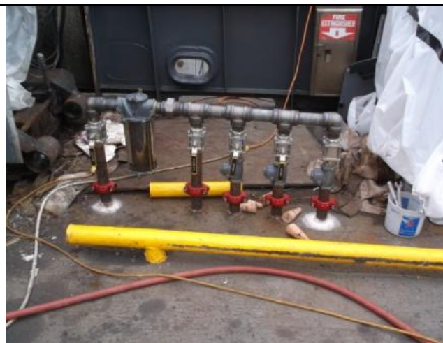
06 New Bilge Washdown Manifold
