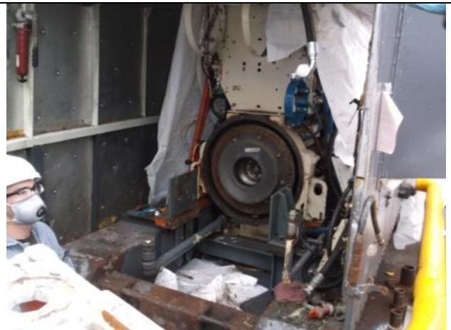
04 Typical Propulsion Engine
