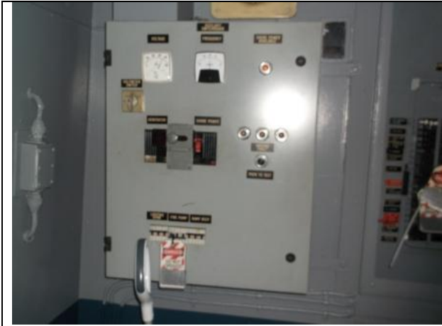
13 Main Switch Gear
