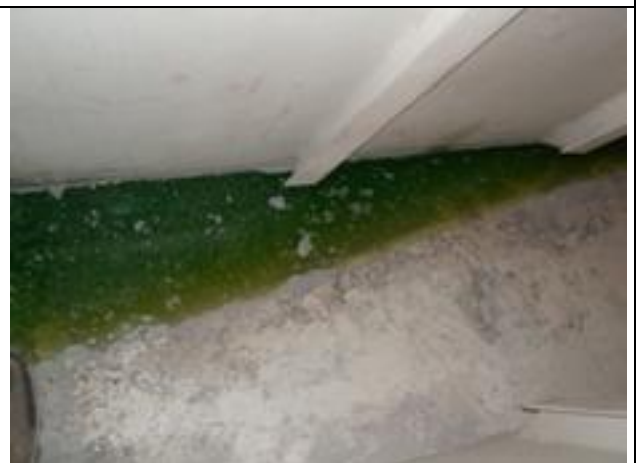
18 Aft Rake Antifreeze in Bilge
