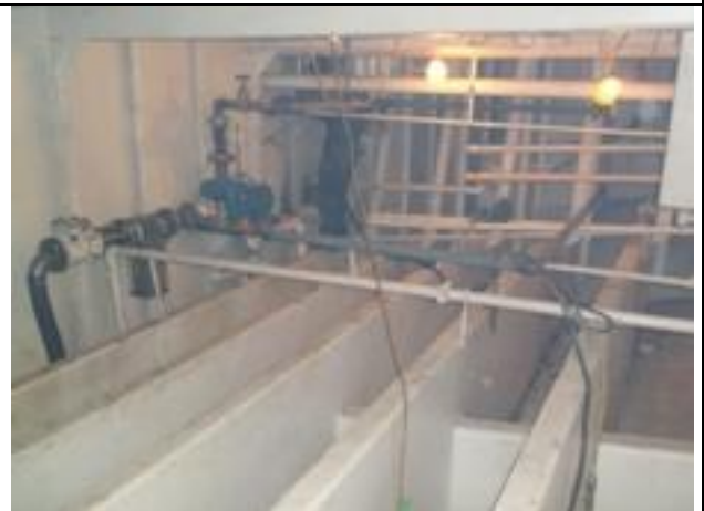
16 Aft Pump Compartment
