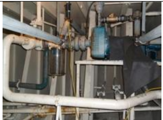
12 Forward Pump Compartment
