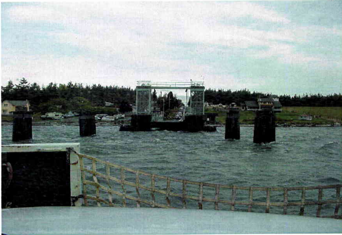
Figure 2.4 - Guemes Island dock, wing walls, and pilings.
