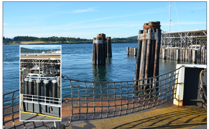
Old pilings at Anacortes terminal; new pilings (inset)
