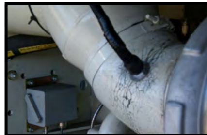
Main Engine #2 – ASF (Injector) Installation
