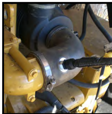
Genset – ASF (Injector) Installation
