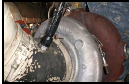
Main Engine #1 – ASF (Injector) Installation
