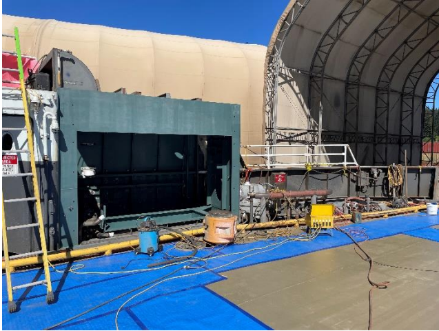
Engine enclosure with first coat of primer
