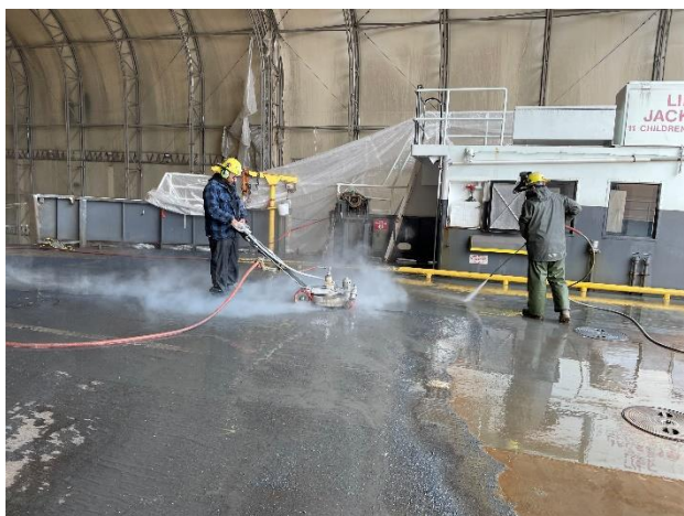
Stripping paint off the car deck.
