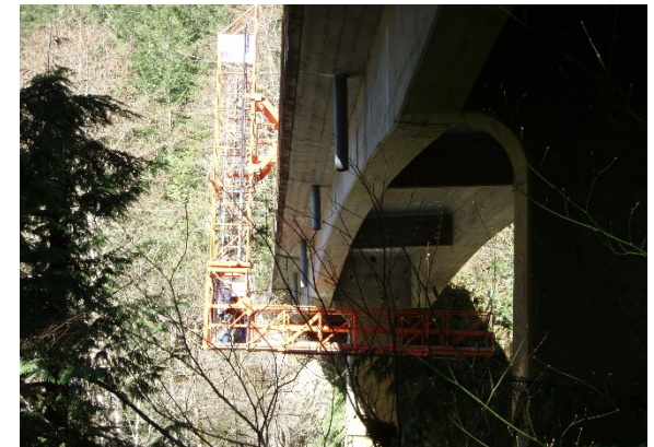
Inspection of Finney Creek Bridge
