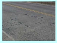
Exposed rebar and cracked, spalling concrete threaten the integrity of the deck and, left unre-
