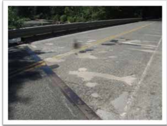
Deck patching on South Skagit Highway's Finney Creek Bridge
