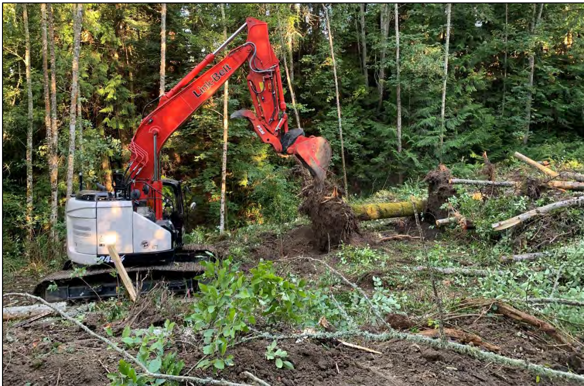
Figure 20: View west, scraping dirt of root wad.
