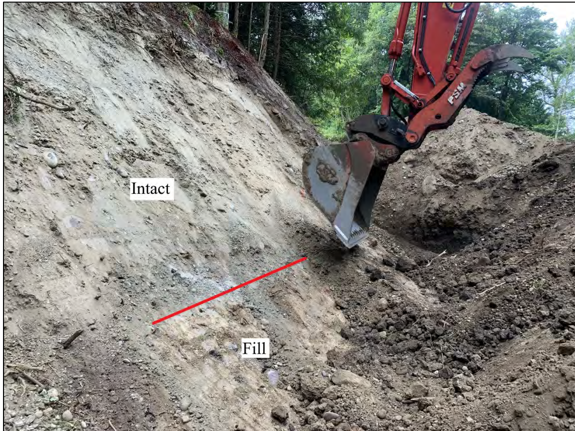
Figure 36: View south, excavating along intact south side slope for new trail grade, remnant fill still evident here as the grade is made.
