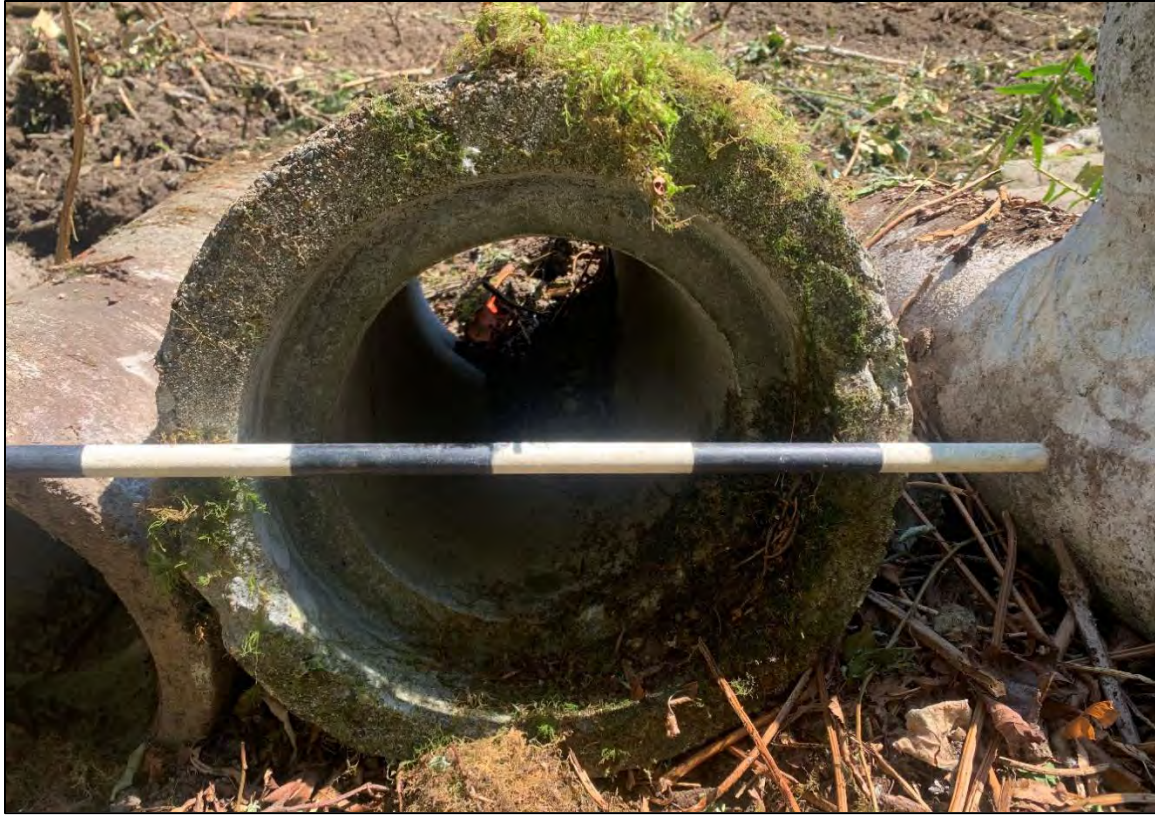
Figure 24: View east, concrete pipe diameter with scale.
