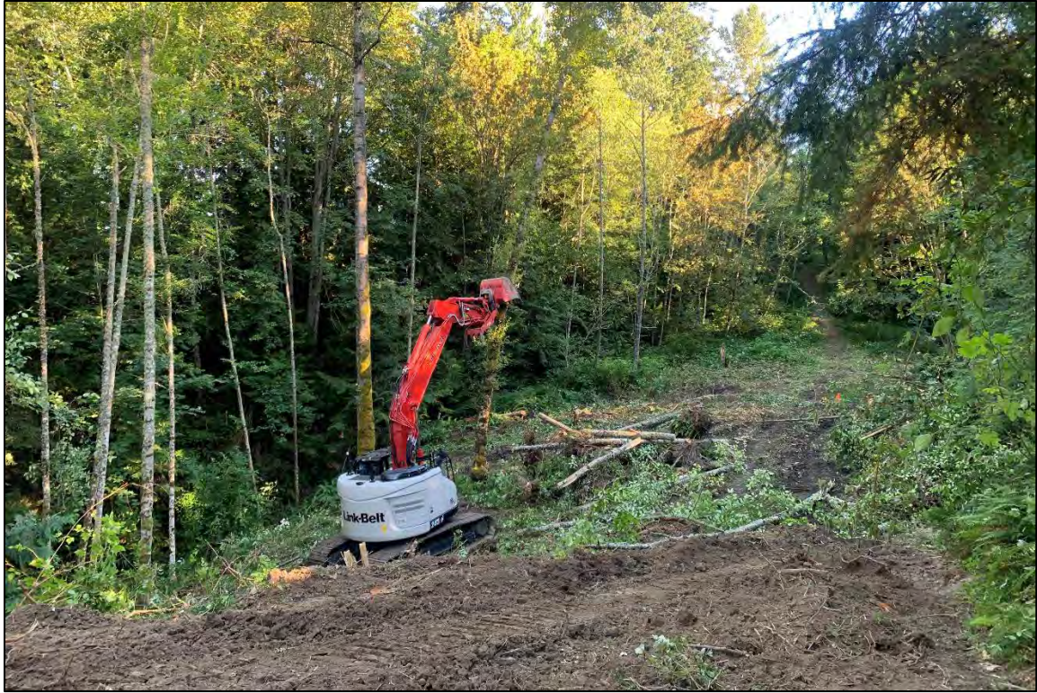
Figure 19: View northwest, felling trees with excavator.
