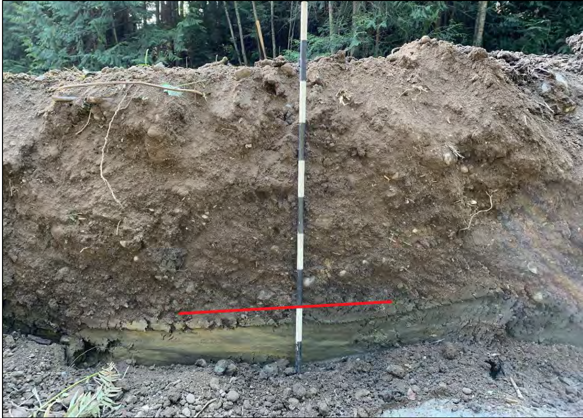
Figure 22: View west, profile in center of culvert, shows silty sand fill over clay fill.
