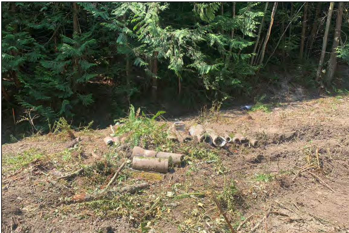
Figure 23: View northwest, concrete pipes exposed in silty sand fill from felled trees.
