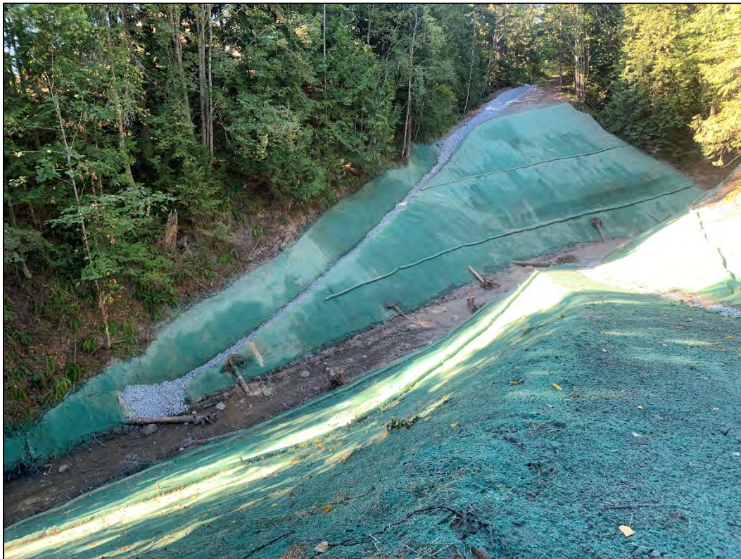
Figure 17: View north, creek at end of Project on August 28, 2020.
