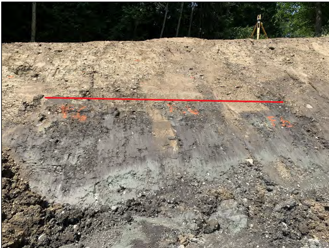
Figure 21: View northwest, north side of creek slope profile, shows silty sand fill over clay fill.
