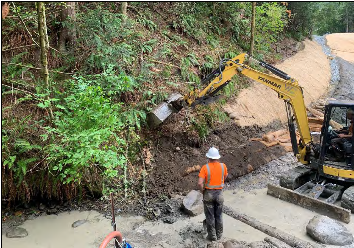
Figure 38: View northwest, excavating along intact slope at downstream end of creek.
