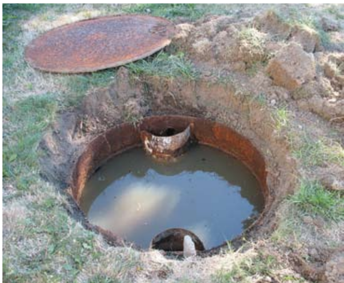
An old, rusted, steel septic tank that has failed. Tanks that fail leak improperly treated sewage and contaminates into our waterways.
