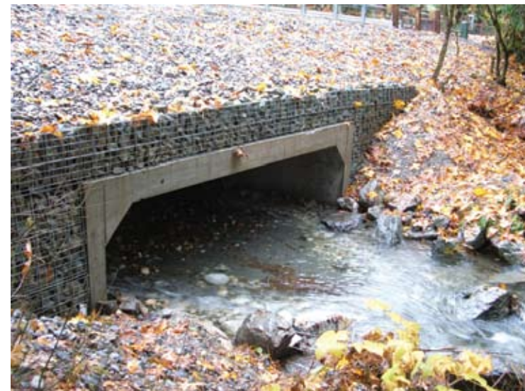
A new culvert at Gravel Creek. This culvert allows fish to swim easily upstream. It is also able to manage the flow of water that may come with rising water levels.
