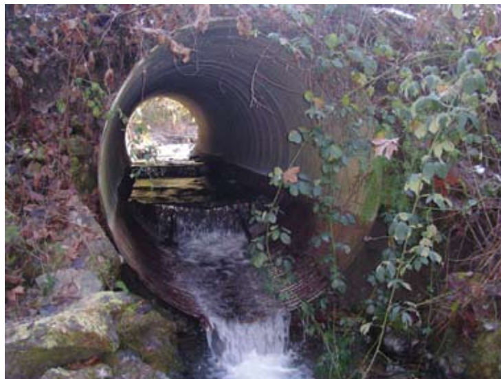
An old culvert at Gravel Creek. This culvert acts as a barrier for fish migrating upstream as the fish are forced to jump up and into the culvert to pass through.
