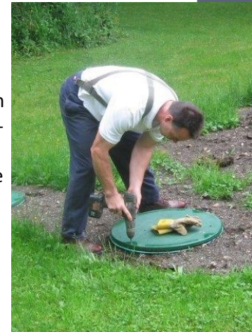
An inspector removing risers to access the septic tank.
