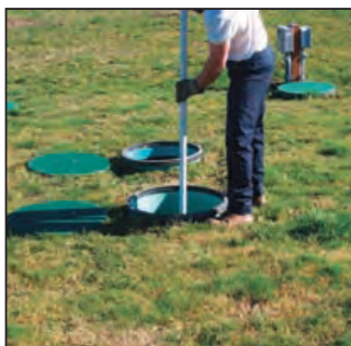
Septic tank inspection in progress
