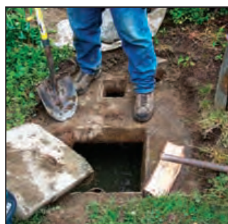
Septic tank baffle screen inspection in progress
