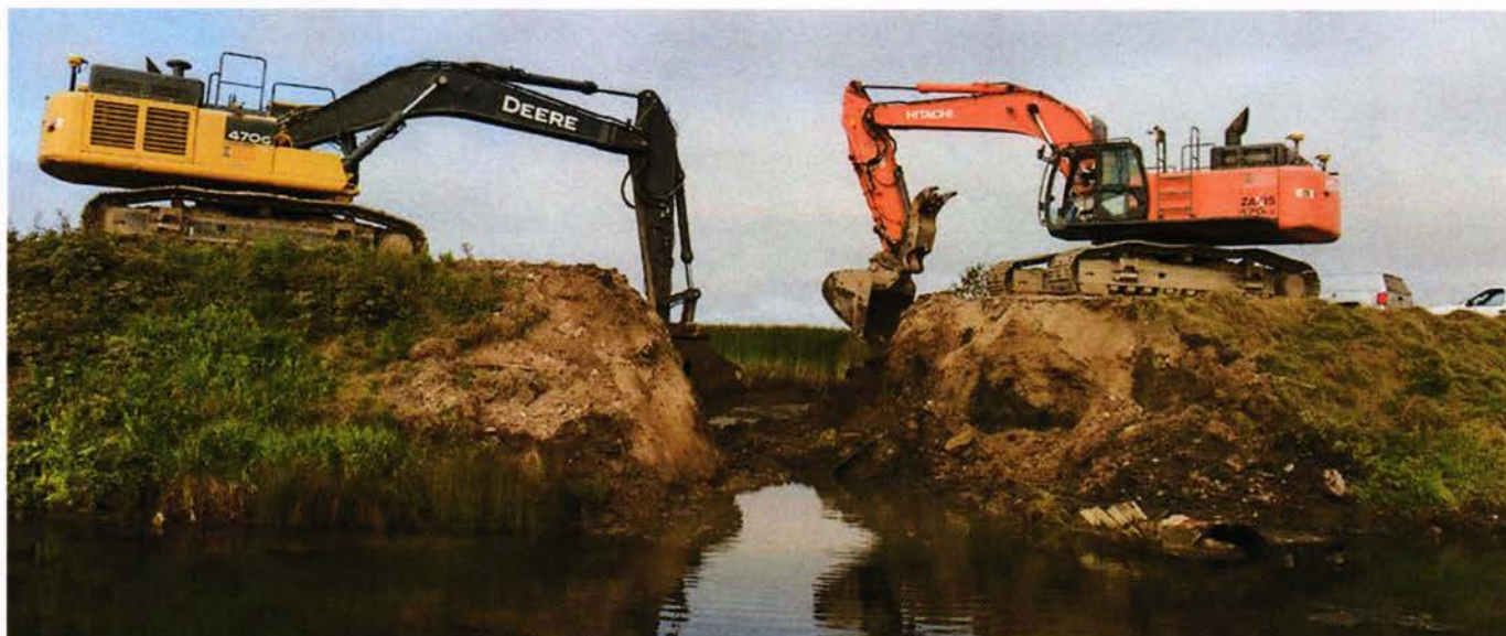
The Fir Island Farm restoration project in the Green Management Group has been completed with 131 acres of estuary habitat restored.
