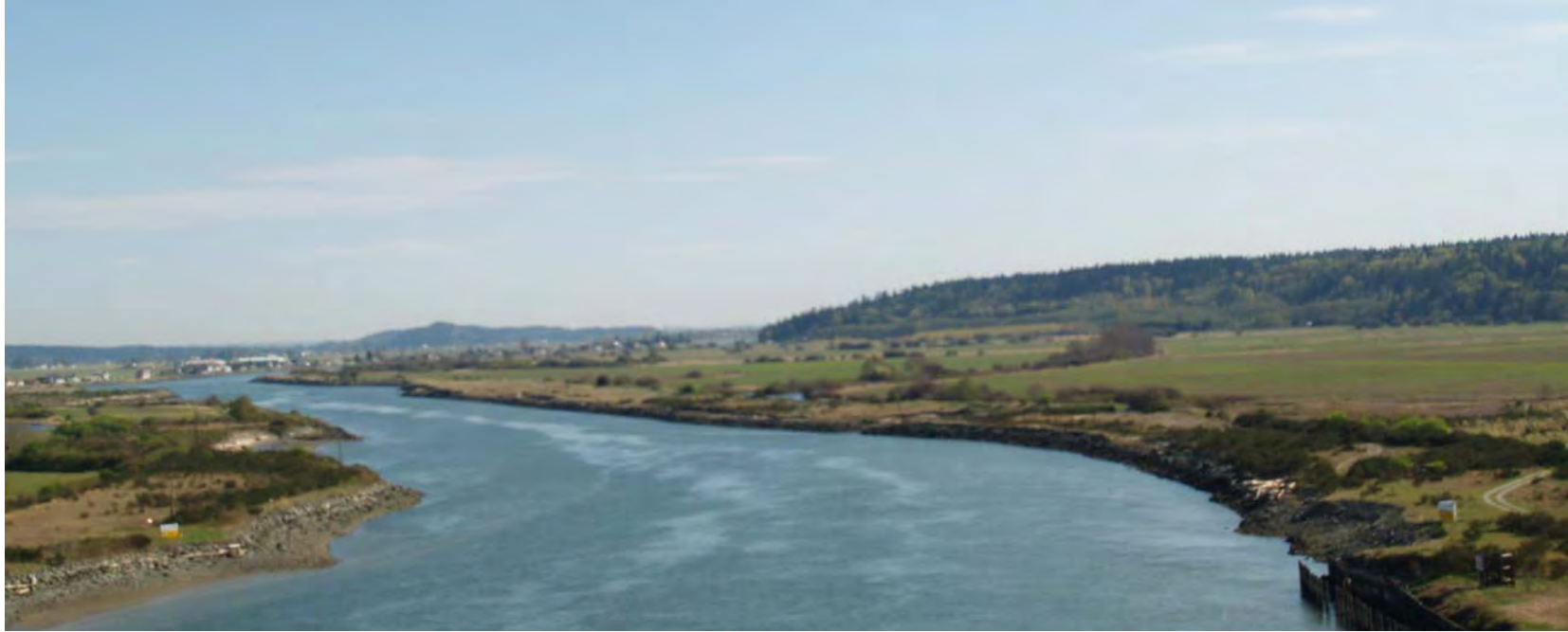
Photo – view to the south of Swinomish Channel from SR-20 bridge to Fidalgo Island
