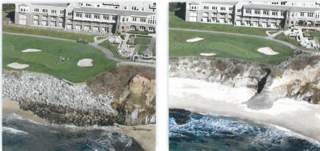
Figure 21. Photo depicting removal of shoreline protective structure. Removal of rock revetment restores access and allows natural bluff erosion at the Ritz Carlton in Half Moon Bay. (Source: California Coastal Records Project )
