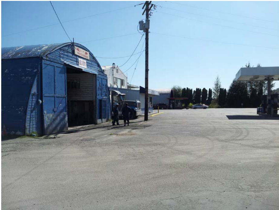
Photo 5. View of the truck washing building and fueling station.
