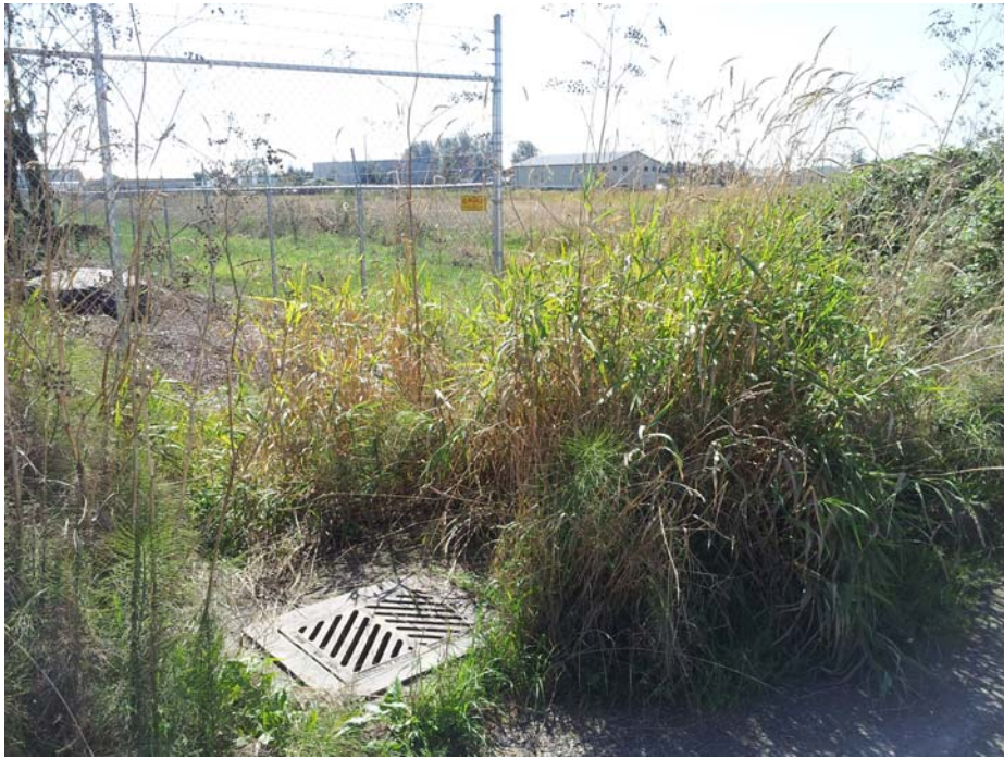
Photo 9. Storm drain on the southern border of the main parcel.
