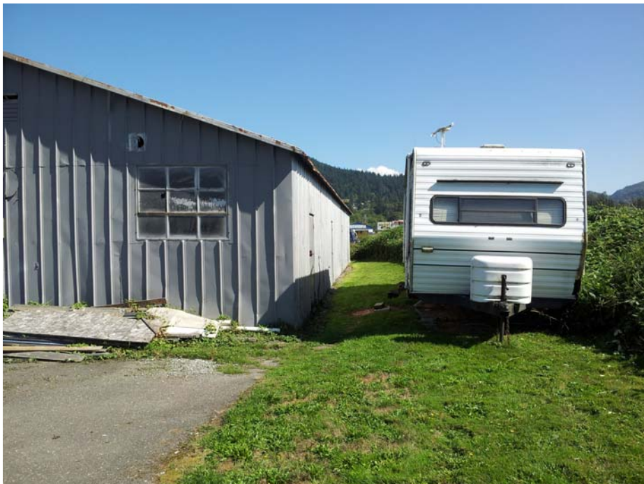
Photo 10. View of the south side of the building on the southern border of the main parcel.
