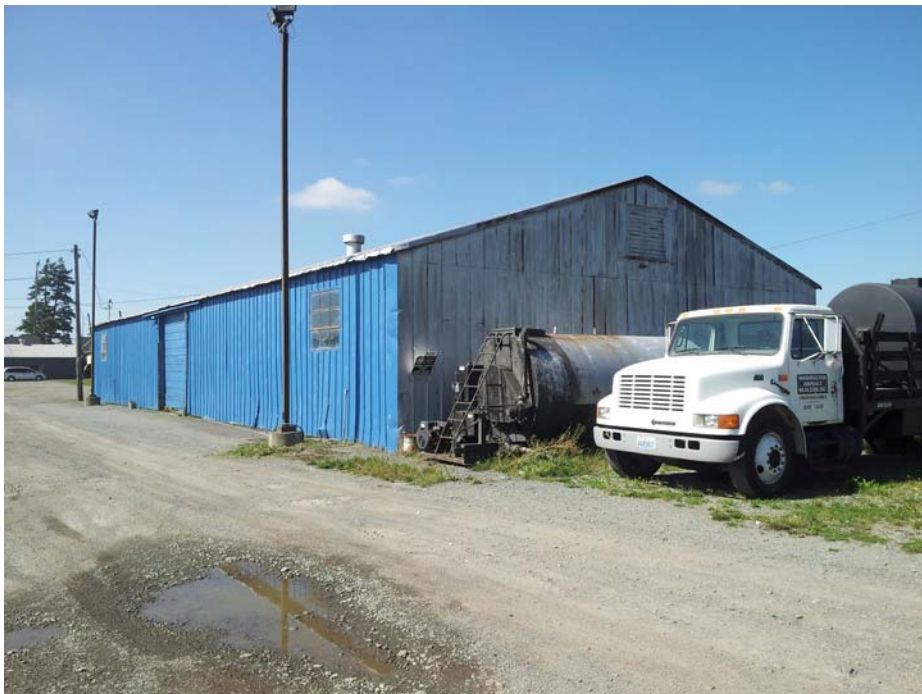
Photo 6. Commercial utility building along northern border of site. Decommissioned storage tank. Paving in very poor condition.
