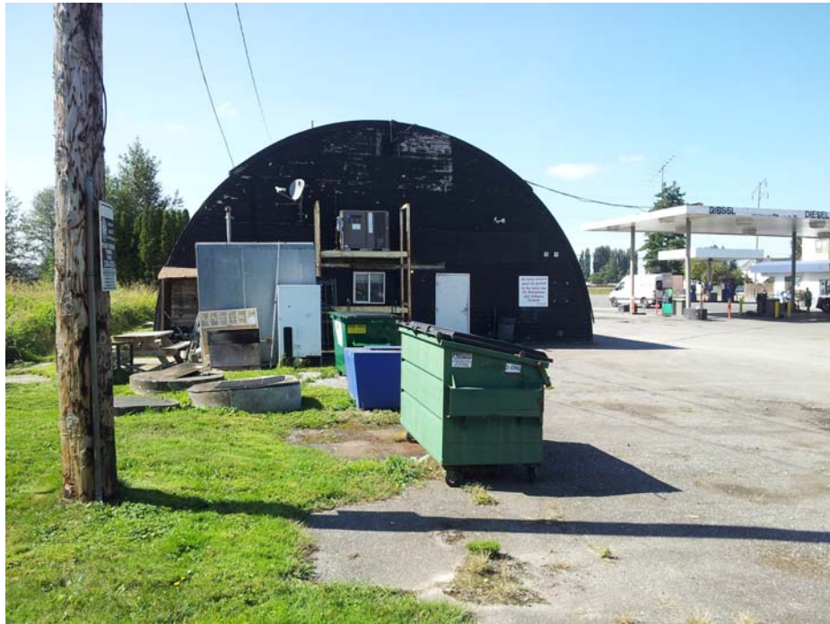
Photo 11. Looking west at the rear of the restaurant.
