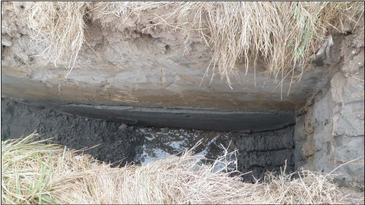
Photo 2. Trench 1, at completion, the profile appeared to be intact.
