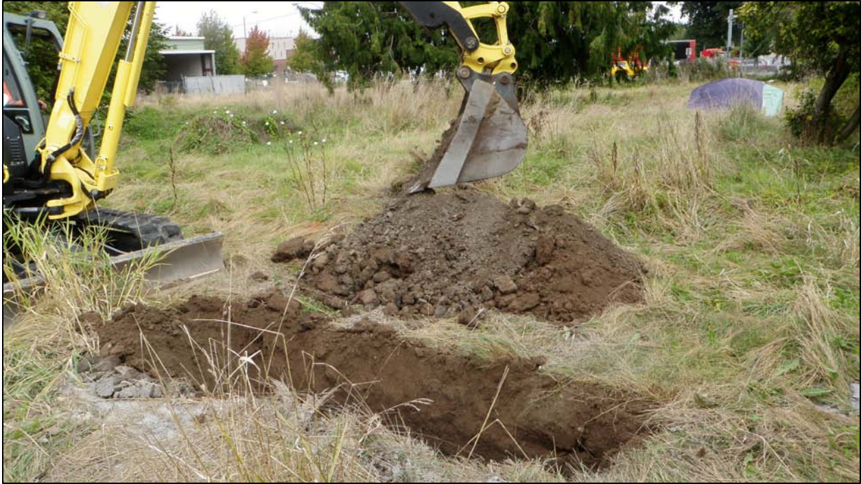
Photo 7. Trench 4 was excavated in the north east portion of the Alf Christianson site.
