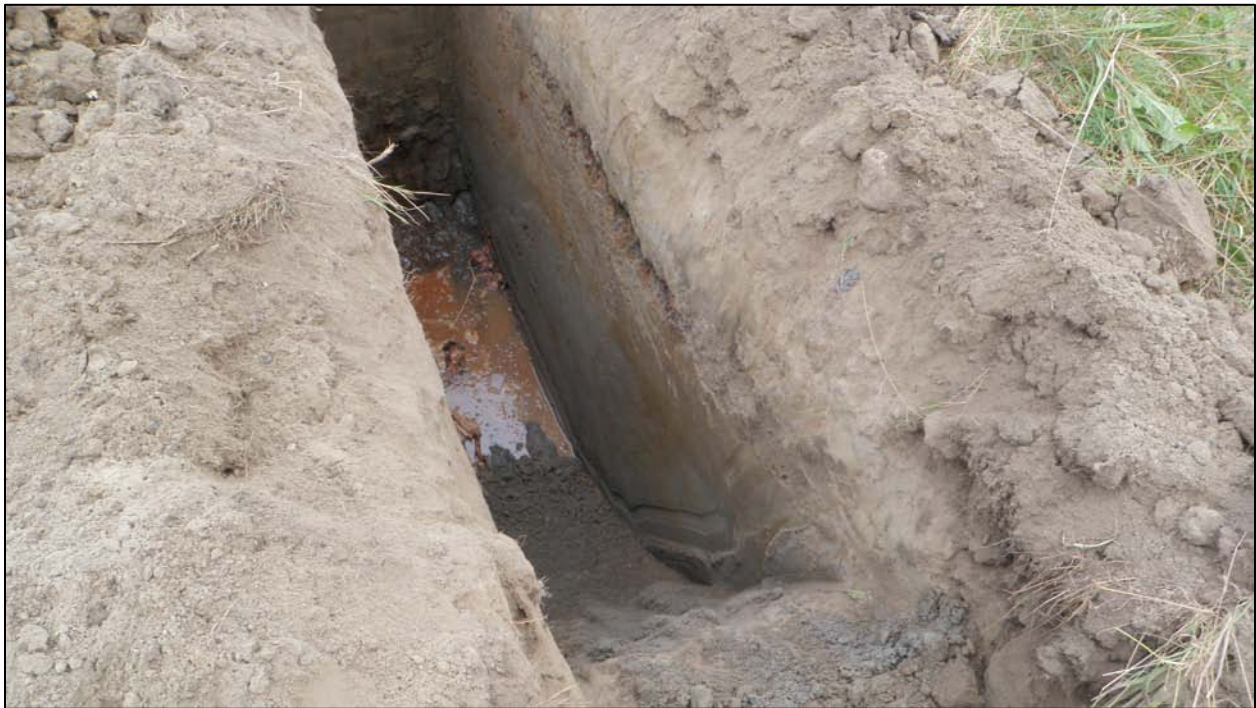
Photo 6. Trench 3 at completion, note the transition from silt to sand midway down and off-colored water.
