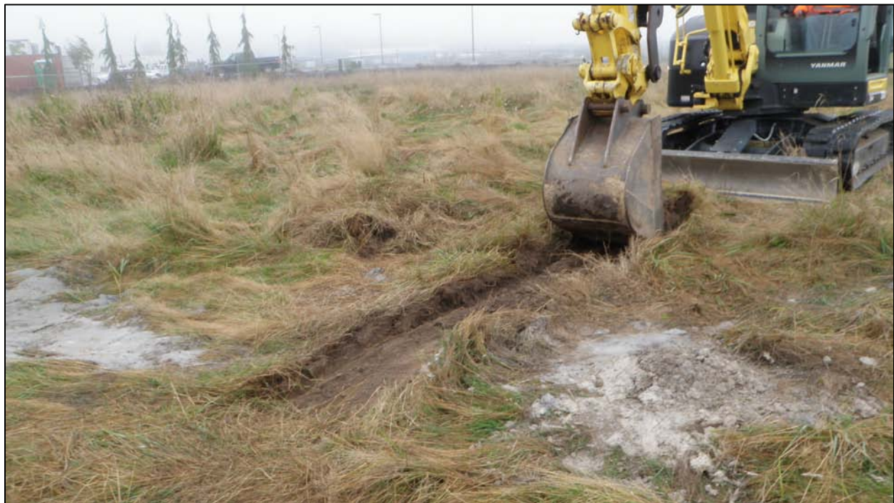
Photo 1. An overview of the Trench 1, looking south east.
