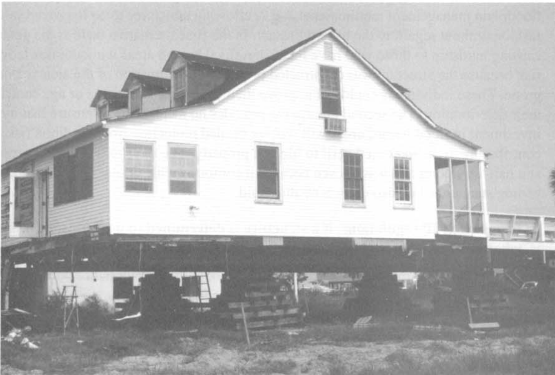
Figure 1. Photograph of a Pre-FIRM structure located on Sullivan's Island, South Carolina which was substantially damaged during Hurricane Hugo. NOTE: The structure has been repaired and is in the process of being elevated to or above the base flood elevation in accordance with NFIP requirements for substantial improvement (Refer to Question No. 9).
