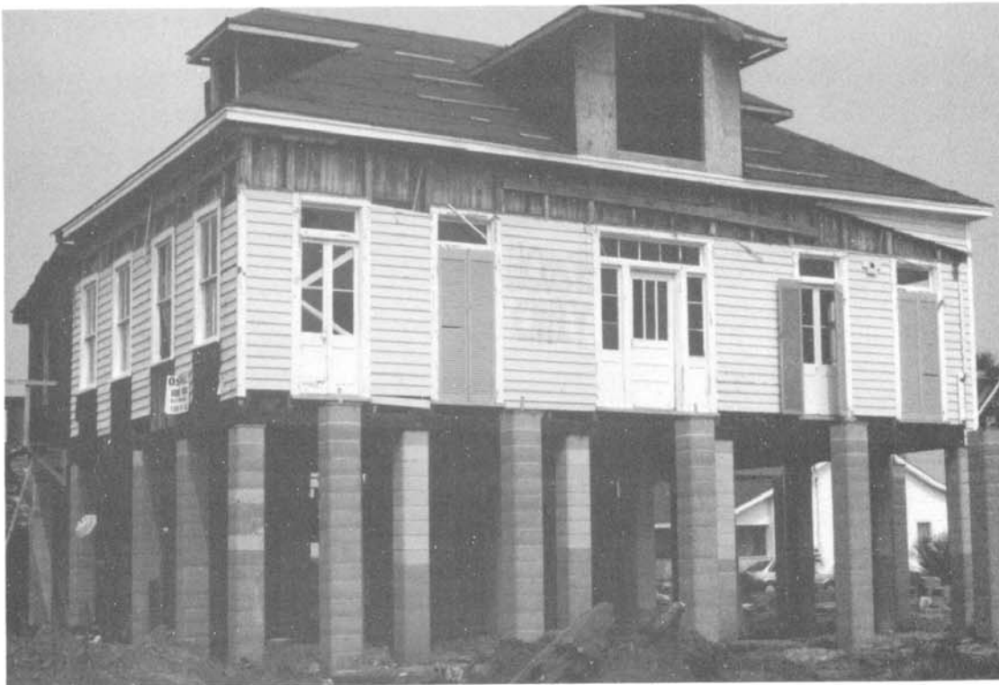
Figure 3. Photograph of a Pre-FIRM structure located on Sullivan's Island, South Carolina which was substantially damaged during Hurricane Hugo. NOTE: The structure is in the process of being repaired and has been elevated to or above the base flood elevation in accordance with NFIP requirements (Refer to Question No. 14).
