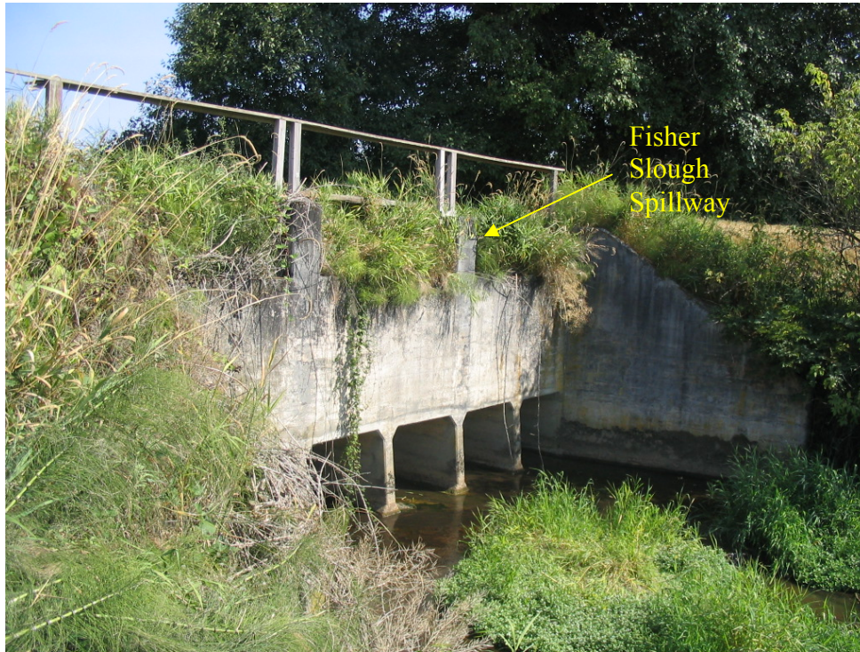
Figure 1. Fisher Slough Existing Emergency Spillway and Existing Big Ditch Culvert Crossing
