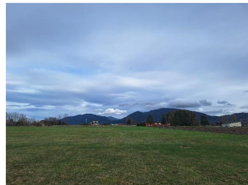
Edison Wastewater Treatment Facility. Photo courtesy of Skagit County Planning & Development
