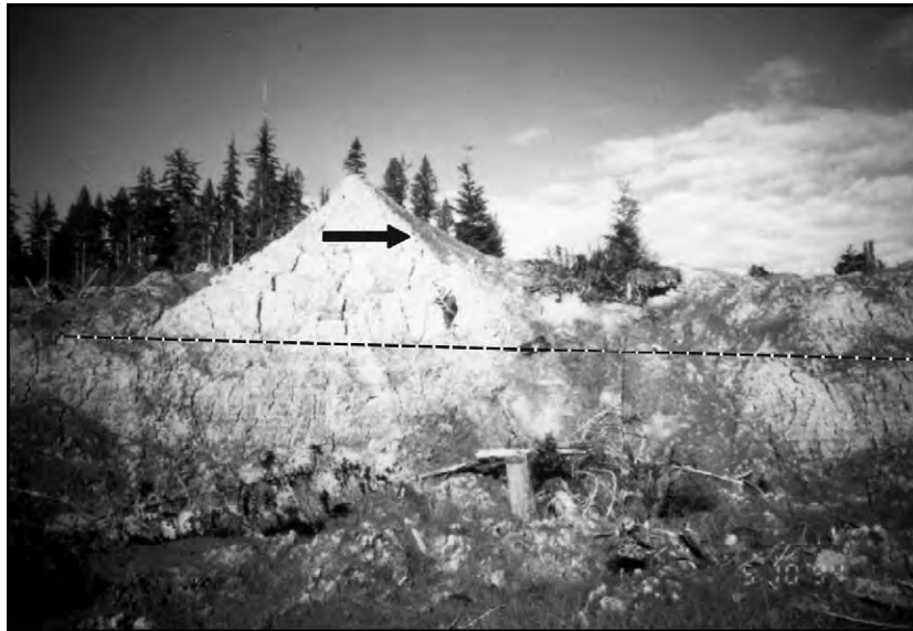
Fig. 15. Prism of glacial marine sediments in the Mink Creek landslide. The prism is part of a transverse ridge that formed by translational movement along a nearly horizontal rupture surface (dashed line). Arrow indicates direction of movement.
