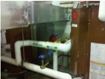
Elementary Gas Fired Water Heater
