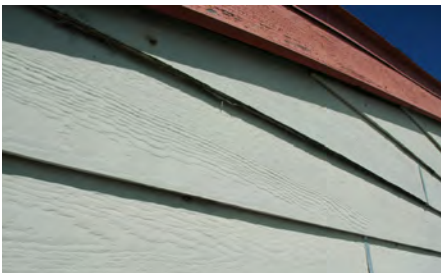
Deteriorated Siding
