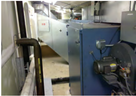
Indoor Gas Fired Air Handling Units
