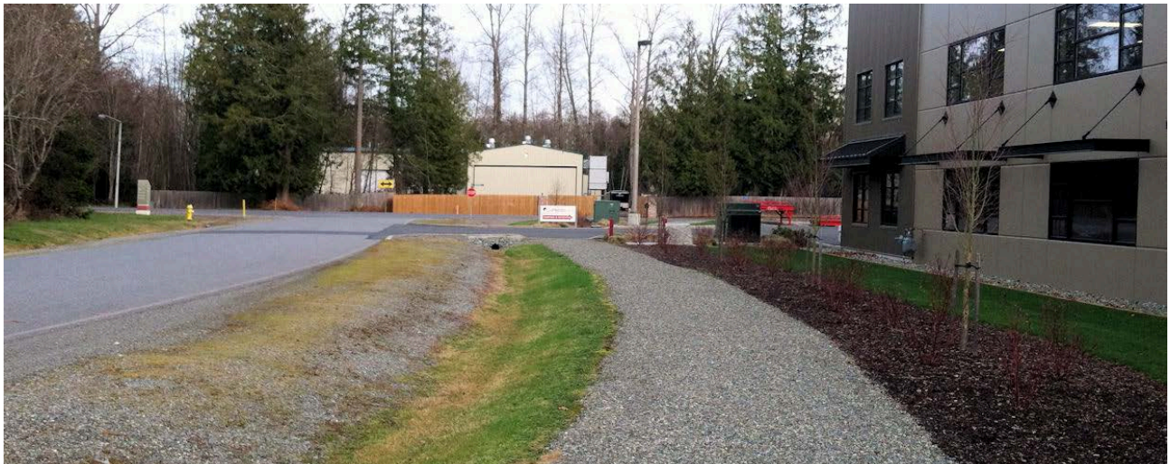
Figure 14.46.420(5). Example street design in the BR-LI zone, including swales and a pathway on one side.
