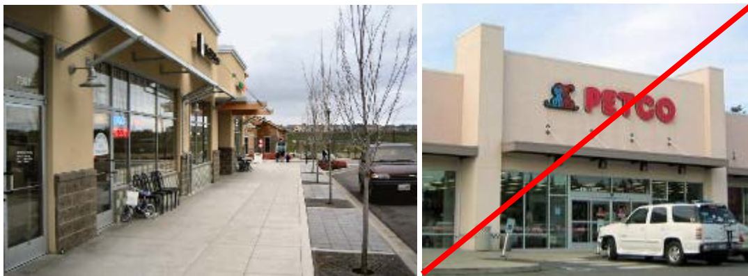
Figure 14.46.536(c). Acceptable and unacceptable stucco examples. The left image uses concrete block near the sidewalk, while the Petco maintains stucco to the base of the façade.
