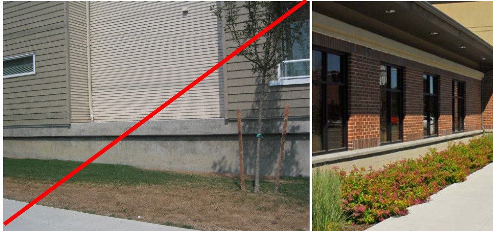
Figure 14.46.540(5)(d). Provide landscaping to screen exposed foundations.
