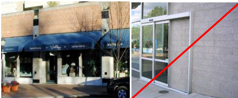
Figure 14.46.536(b). Acceptable and unacceptable concrete block examples. The left example uses a mixture of split-faced colored concrete block and smooth-faced concrete block, together comprising just under 50% of the whole façade. The large expanse of smooth-faced concrete block on the right is not desirable for Bayview Ridge façades.
