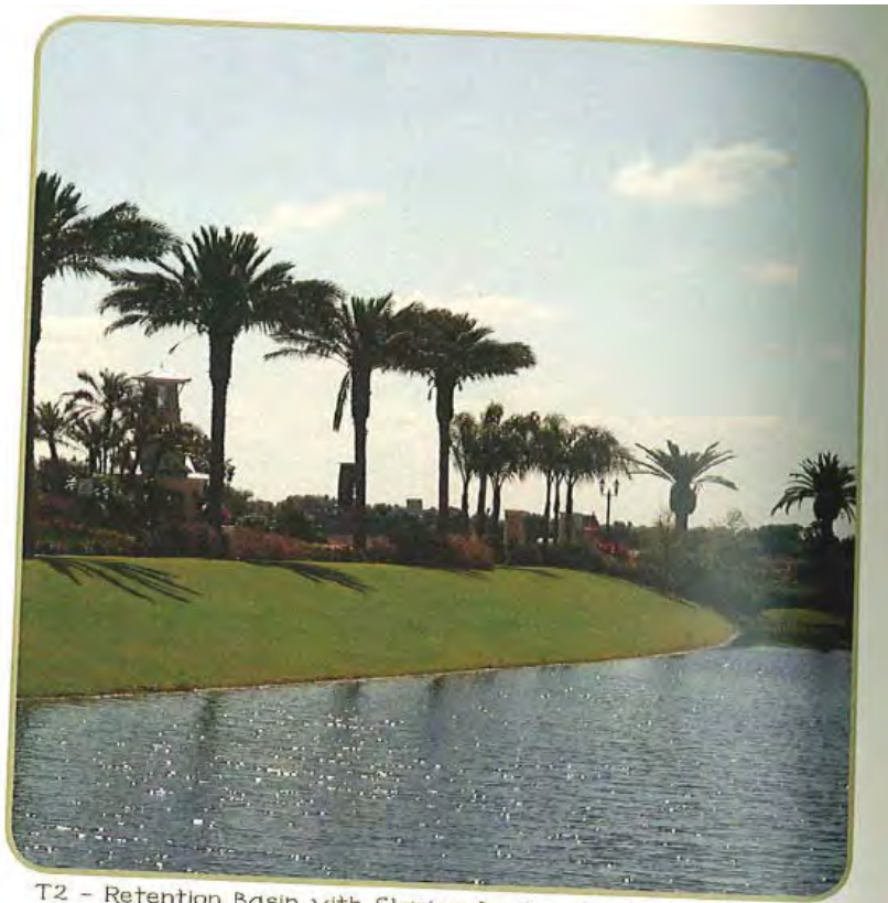
T2 - Retention Basin with Sloping Bank - Apollo Beach, FL
