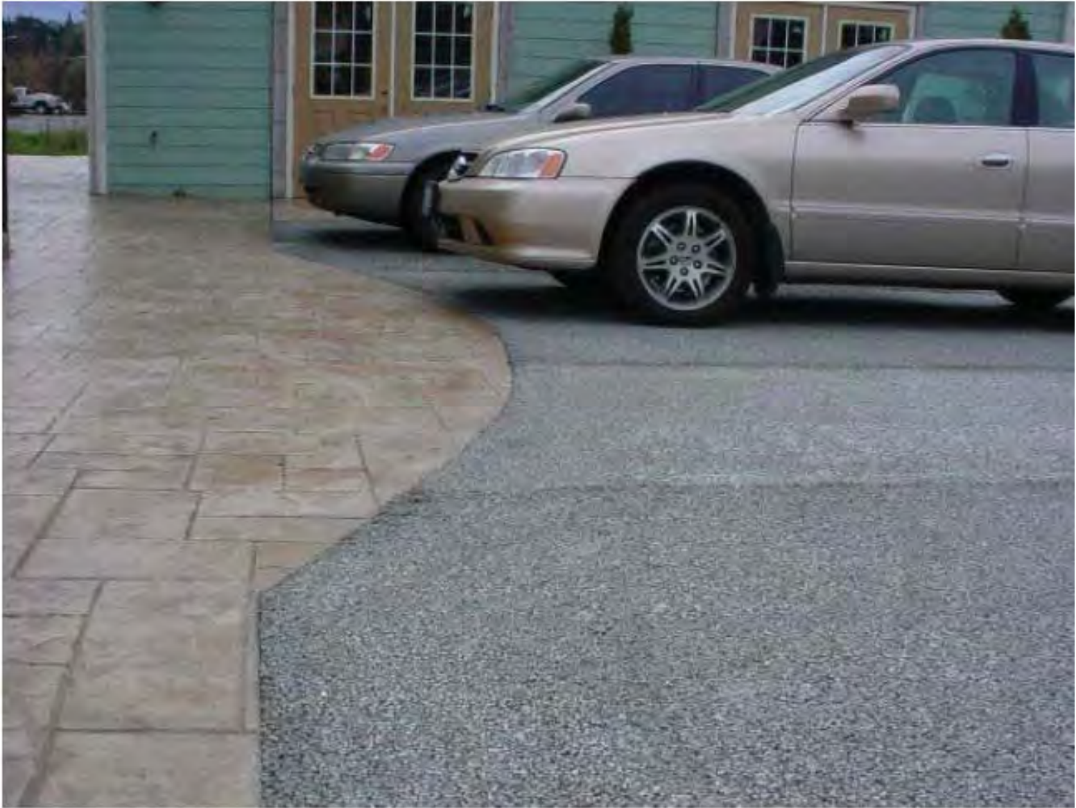
Stamped and Permeable Concrete Pavement Photo by Curtis Hinman (2005 LID Manual)
