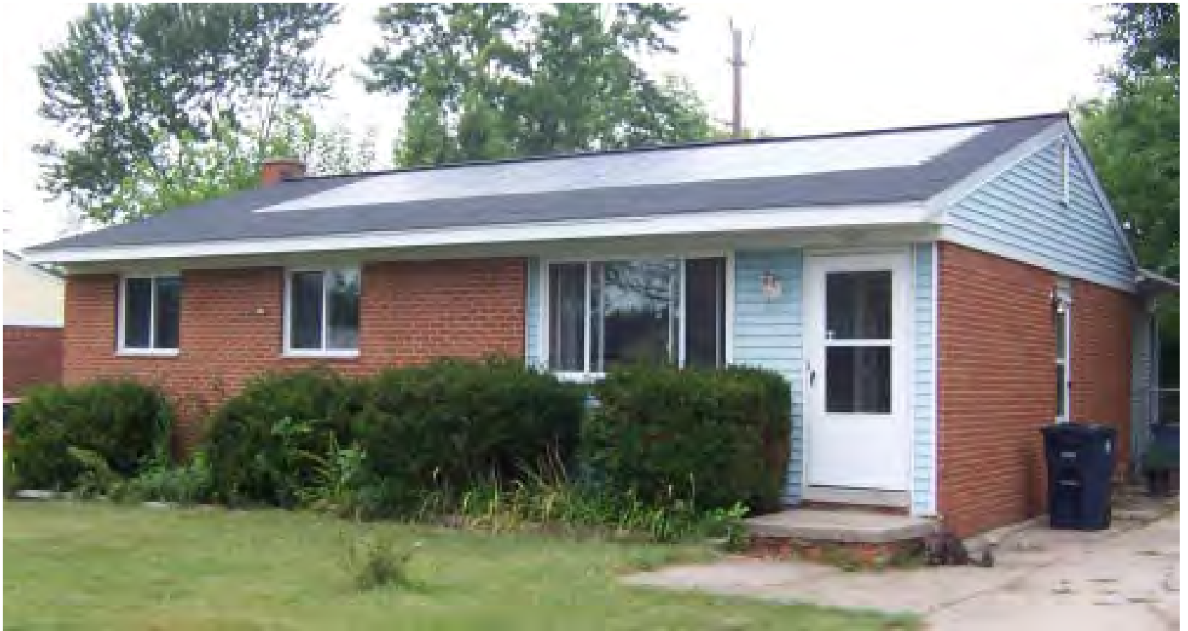
Individual Solar PV
