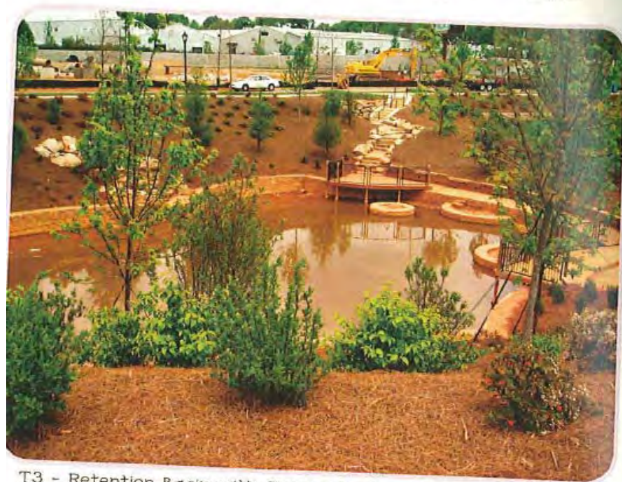
T3 - Retention Basin with Sloping Bank - Glenwood Park, GA
