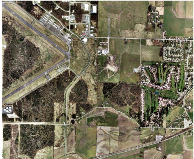
Figure 1. The boundaries of the Subarea reflect major industrial/commercial property ownerships, existing land use, and topography. The Avon-Allen Road and a steep hillside form the boundary on the east. State Route 20 (SR 20) and Ovenell Road bound the Subarea to the south, with the Farm to Market Road on the west and the Port of Skagit County ownership, Josh Wilson Road, and a steep hillside on the north.
