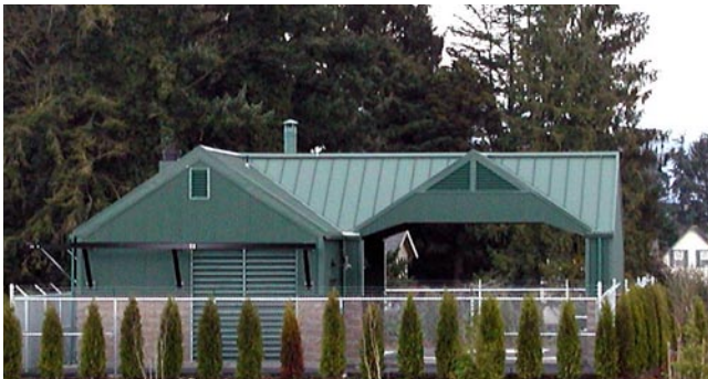
Sewer Pump Station on Peterson Road near Avon-Allen
