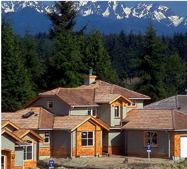
Figure 3 provides a view of the existing development in the Bayview Ridge Subarea.
