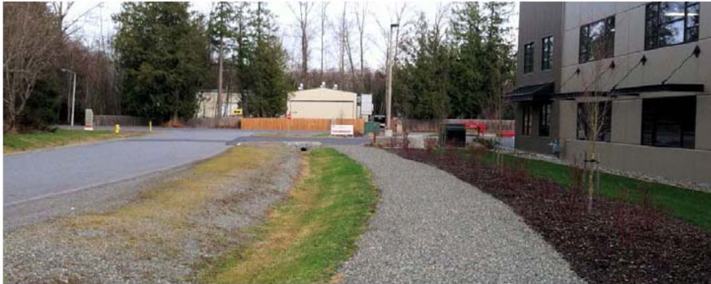
Figure 14.46.420(5). Example street design in the BR-LI zone, including swales and a pathway on one side.
