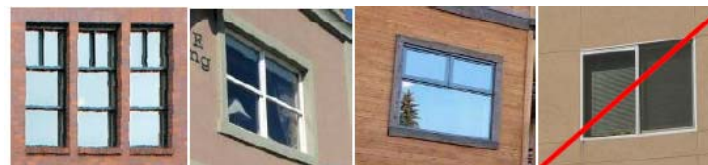
Figure 14.46.530(5)(b). Acceptable and unacceptable (far right image) window design on upper floors. Note that the windows in the brick building on the left are recessed from the façade. The windows in the middle images include trim. The image on the right includes no trim or recess/projection, and thus would not be permitted.
