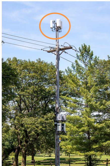
Figure 2 Small Wireless Facility
