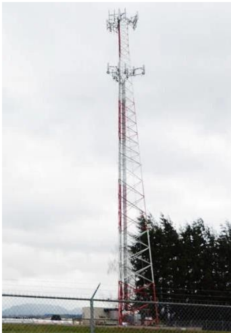
Figure 1 Macro Cell Tower
